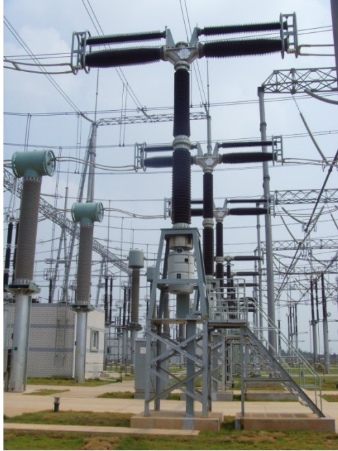
Fig.1.1: LW15-550 outdoor H.V.A.C porcelain SF 6 circuit breaker from XIAN XD high voltage switchgear Co., Ltd.
