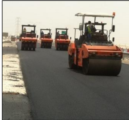
Figure 37. Paving of PG76-10E and PG76-22S asphalt concrete mixtures.
