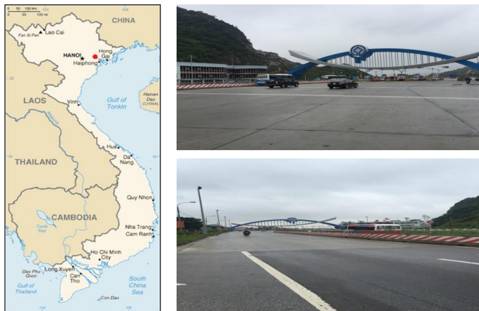
Figure 9. 5 No 18 Uong Bi – Ha Long Highway
