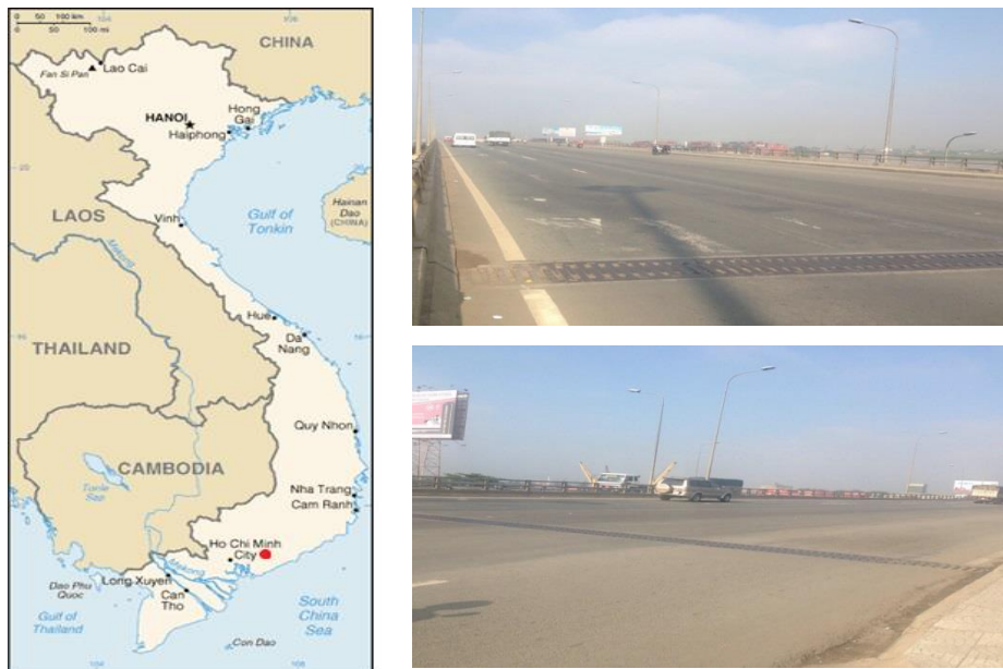
Figure 9. 7 New Dong Nai Bridge
