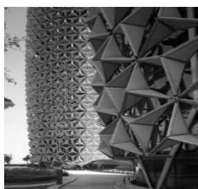
Figure 2. Al Bahar Towers
