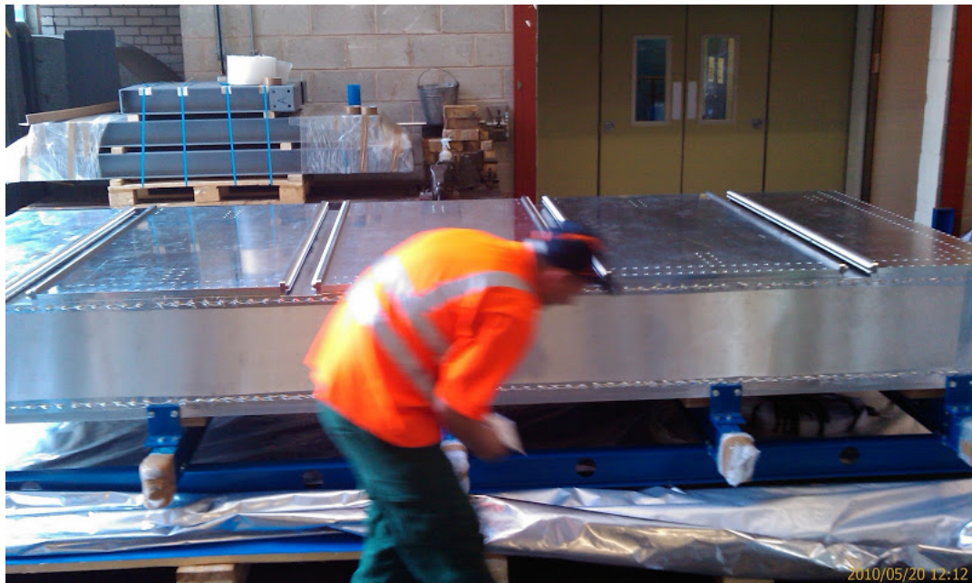
Figure 3.18: A completed module in preparation to be shipped.
