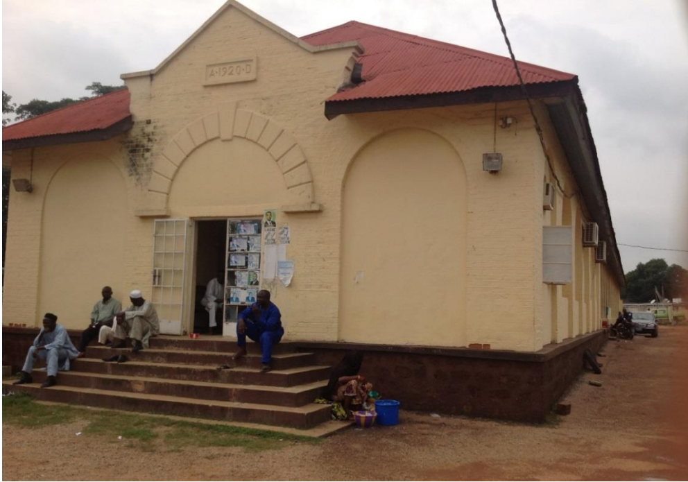
Figure 77: 1920 Court house Kaduna – front view (Picture taken by Author in 2013)
