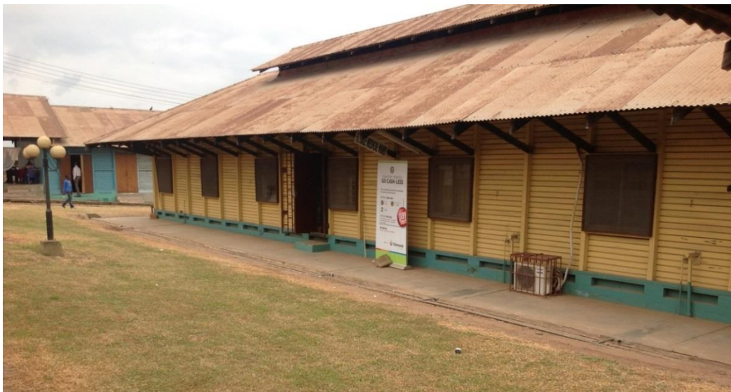
Figure 83: 1926 General Hospital Abeokuta with mosquito proofing (Picture taken by author in 2013)
