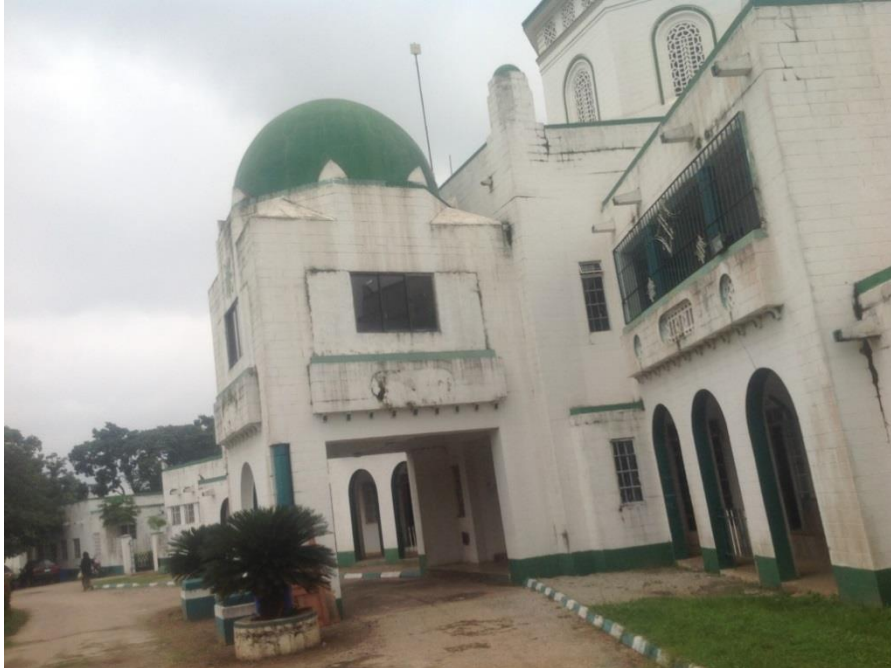
Figure 65: Regional architecture features of Lugard memorial council chamber, 2013 (Picture taken by author)
