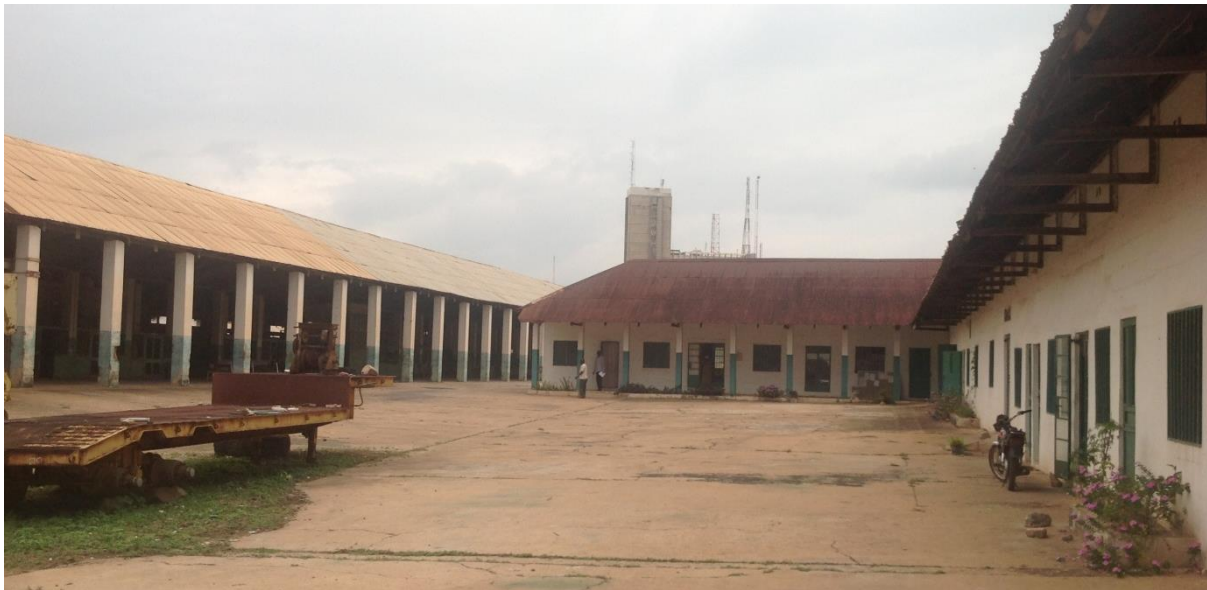
Figure 50: PWD maintenance yard and offices in Kaduna (Picture taken by author in 2013)
