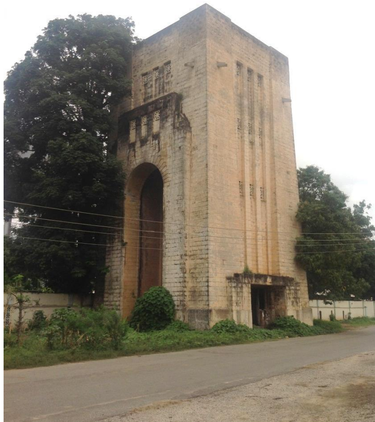
Figure 171: Water Tower Kaduna, designed by Thomas Scott (Picture taken by author in 2013)
