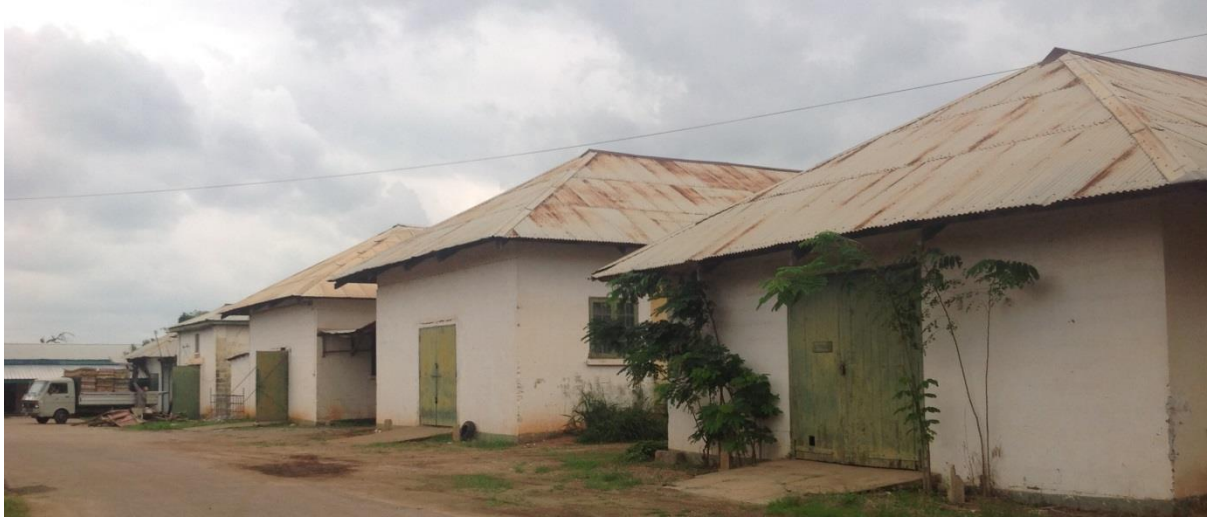
Figure 49: PWD yard stores in Kaduna [Picture taken by author in 2013]
