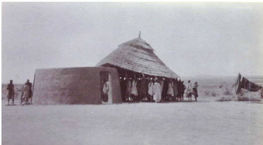
Figure 111: A circular Zaure under construction with roof being hoisted
