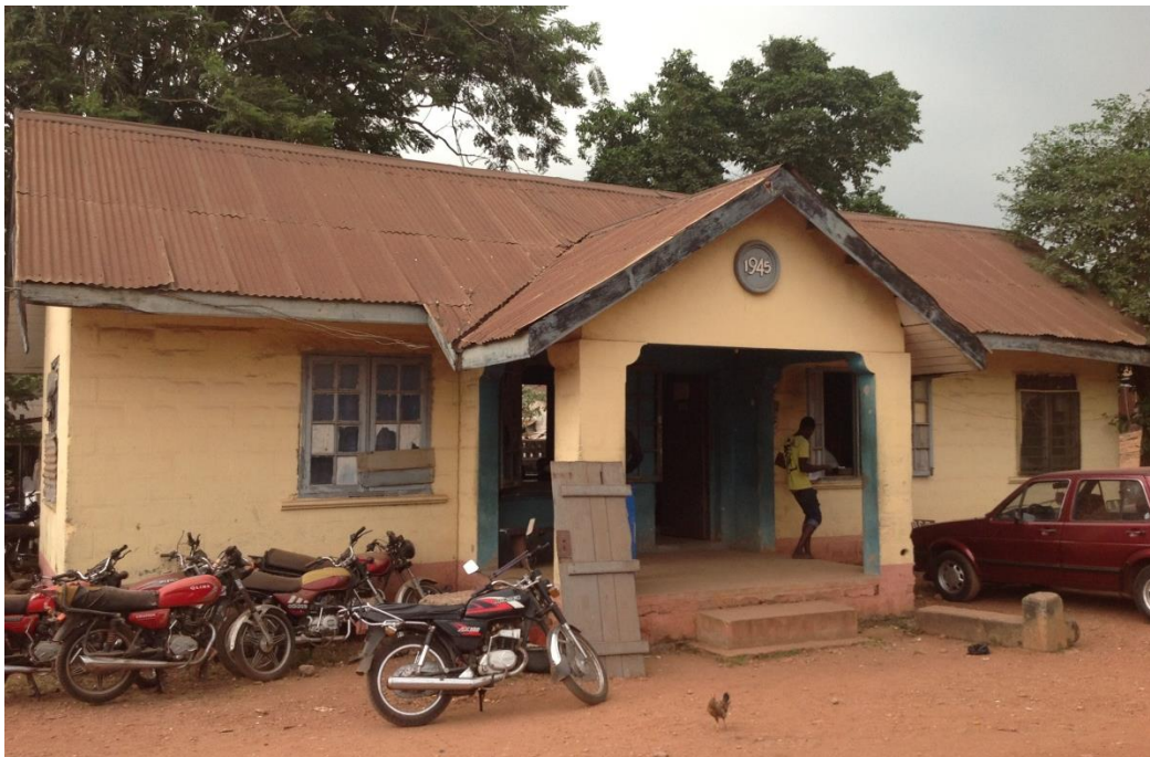
Figure 79: 1945 Police Station Abeokuta (Picture taken by author in 2013)
