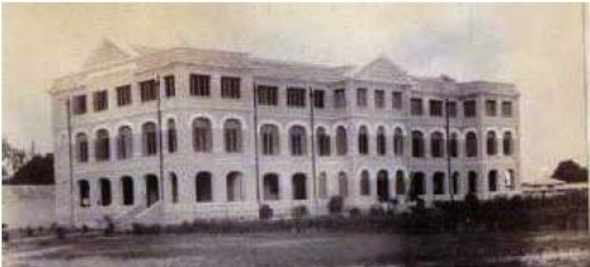
Figure 60: Government house Lagos before front entrance extension 381
