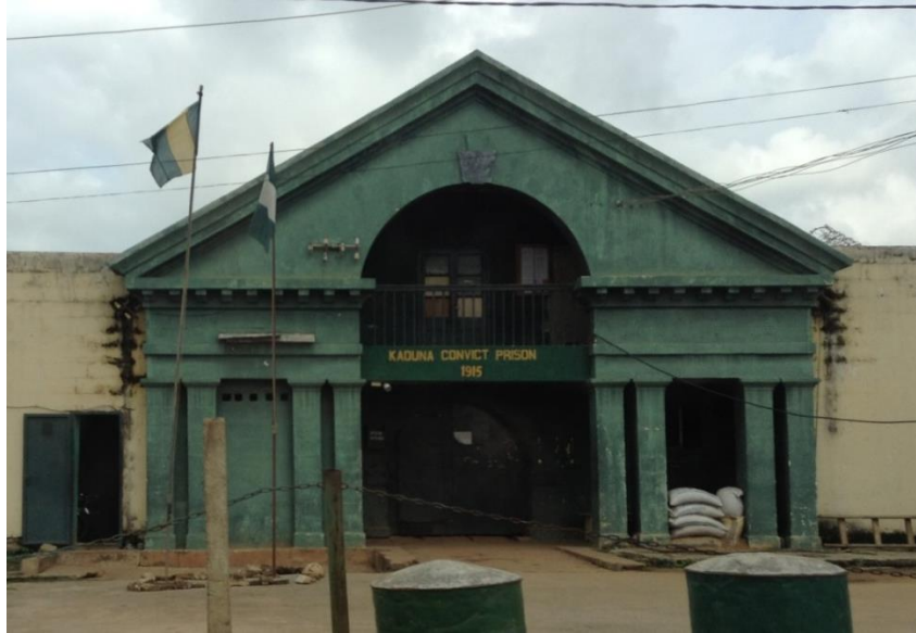
Figure 92: 1915 Kaduna Convict Prison main entrance (Picture taken by author in 2013)
