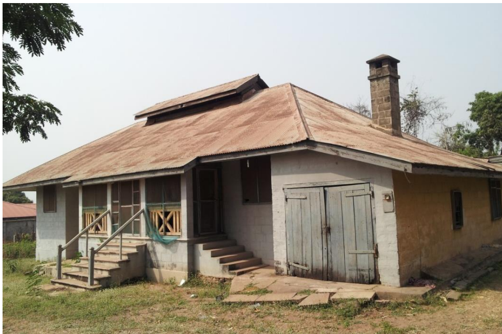
Figure 84: c.1920 Engineer’s quarters Abeokuta with mosquito proofing and roof vent (Picture taken by author in 2013)
