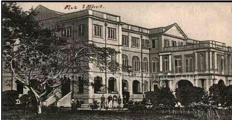
Figure 61: Government house Lagos with extended front entrance porch 384
