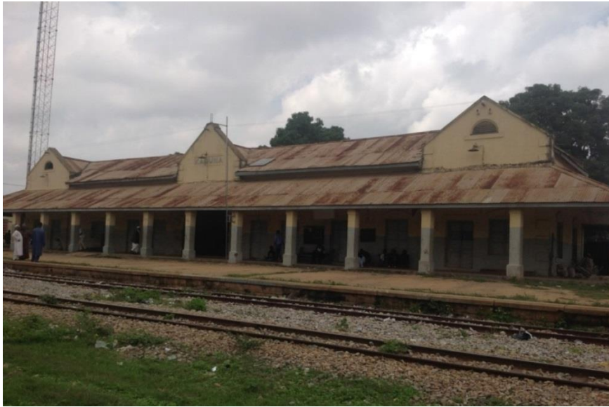
Figure 97: 1920 Railway Station Kaduna (Picture taken by author in 2013)
