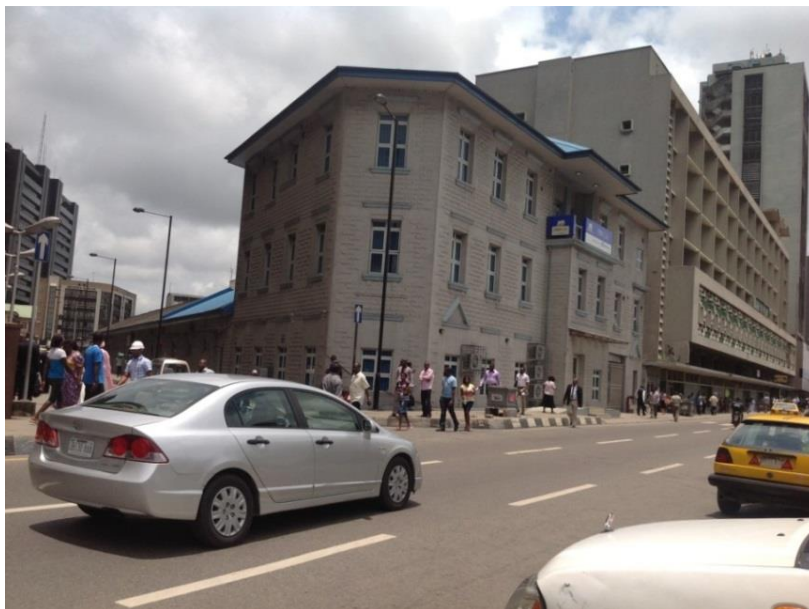
Figure 104: c 1920 Post Office, Marina Lagos, in 2013 488
