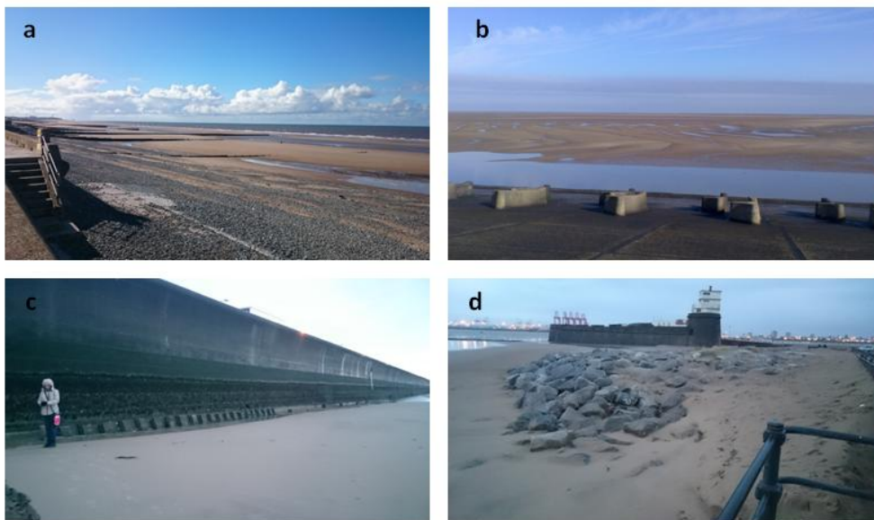
Figure 2.11: Examples of hard engineering schemes in the northwest UK (a) groyne field, Cleverlys, (b) revetments, north Wirral coast, (c) Seawall at New Brighton northwest UK (Person pictured for scale), (d) rock armour exposed at New Brighton marine lake (North Liverpool visible in the background).
