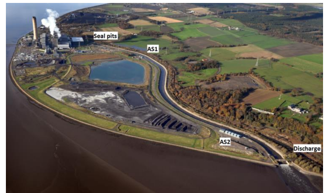
Figure 3. Aerial view of the whole station from the east
