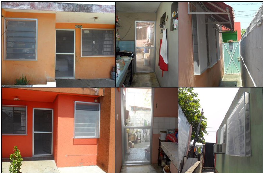
Figure 45. Photographs show the long-lasting insecticide-treated screens (LLIS; Duranet®) mounted on aluminum frames and fixed to windows and external doors of treated houses in Merida, Mexico.
