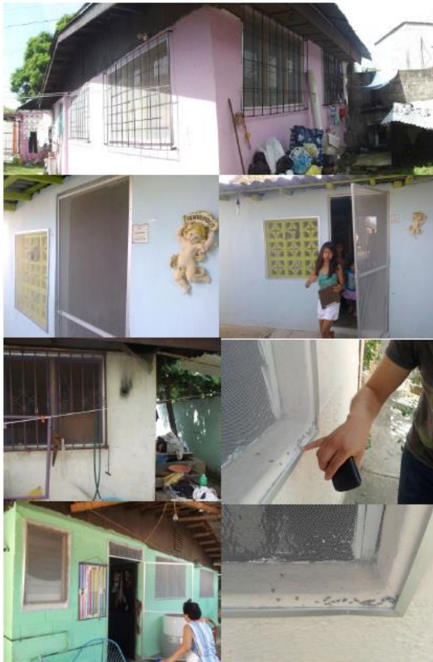
Figure 33. The LLIS intervention (Duranet®) set as framed mosquito screens on windows and external doors of treated houses in Ciudad Renacimiento, Acapulco, Mexico.
