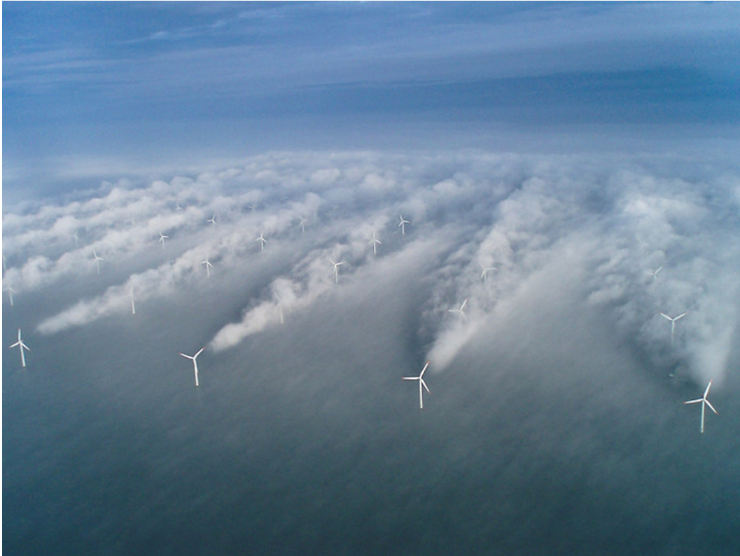
FIGURE 1.8: Picture of air wakes behind wind turbines, Horns Rev windfarm, Denmark. ( www.noaanews.noaa.gov , 2011 [53], credit to Vattenfall)
