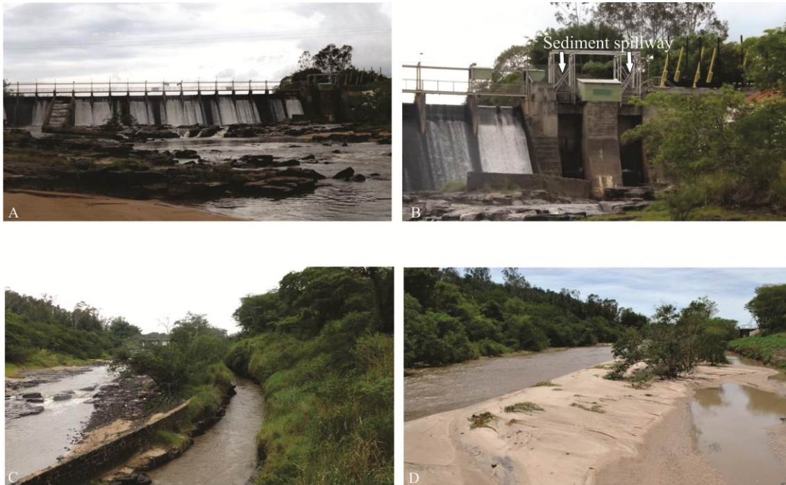
Fig. 3. (A) View of Quatiara hydroelectric, located upstream of the reaches, (B) view of the dam showing the sediment spillway, (C) channel downstream of the dam, and (D) volume of sediments mobilized by the opening of the spillway (available from http://www.nossalucelia.com.br/n7745.html ).
