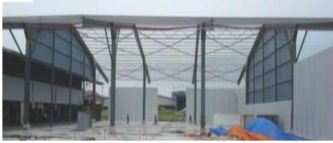
(a) UHPFRC portal frame in Malaysia
