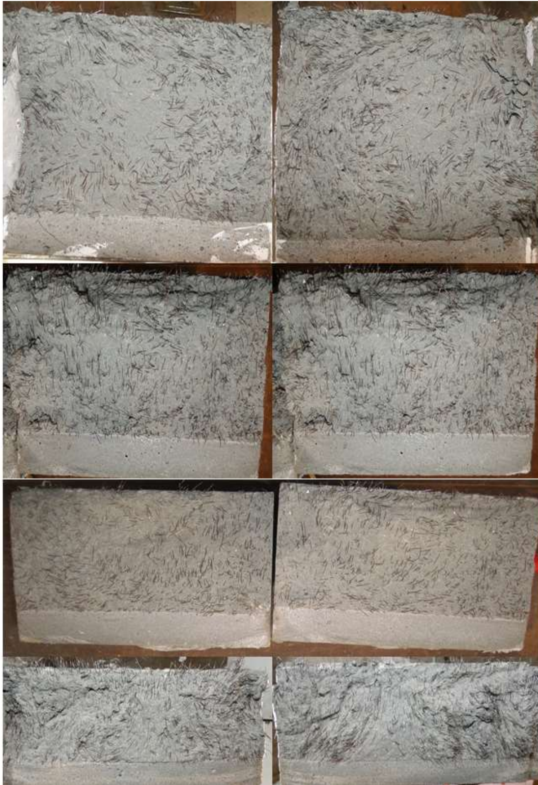
Figure 3.12: Crack location of beam specimen with different thicknesses.
