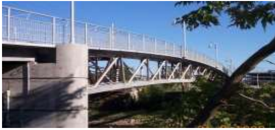
(a) Sherbrooke footbridge in Canada
