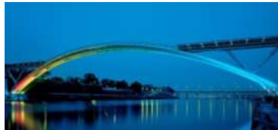
(h) Peace footbridge in South Korea
