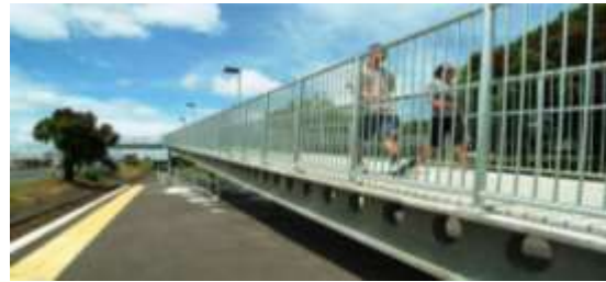
(f) Papatoe footbridge in New-Zealand
