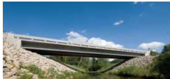
(j) Wapello County bridge in USA
