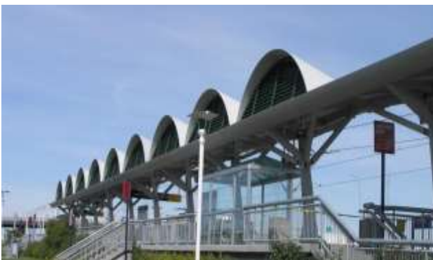
(c) Shawnessy LRT Station in Canada
