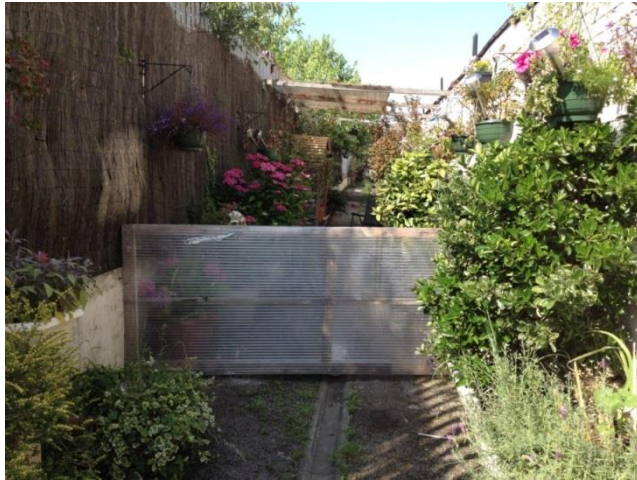
Figure 9.11 CMP have erected an informal boundary to segregate the alleyway
