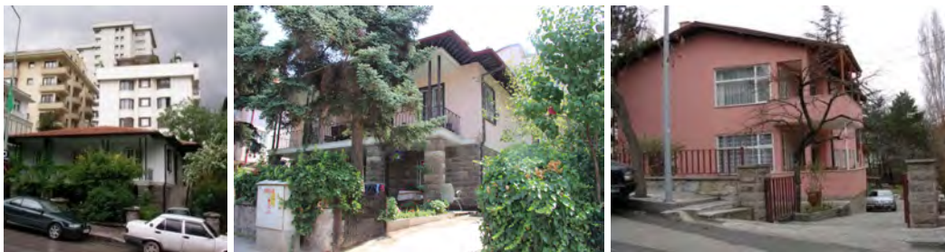
Figure 6.11 Examples of the existing 14 Mayıs Houses (the photo on the left shows how the area was occupied by high-rise apartment buildings which replaced the low-rise, medium-coverage existing housing tissue)
