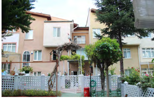
Figure 8.16 Continuous façade pattern and openings in Case IV
