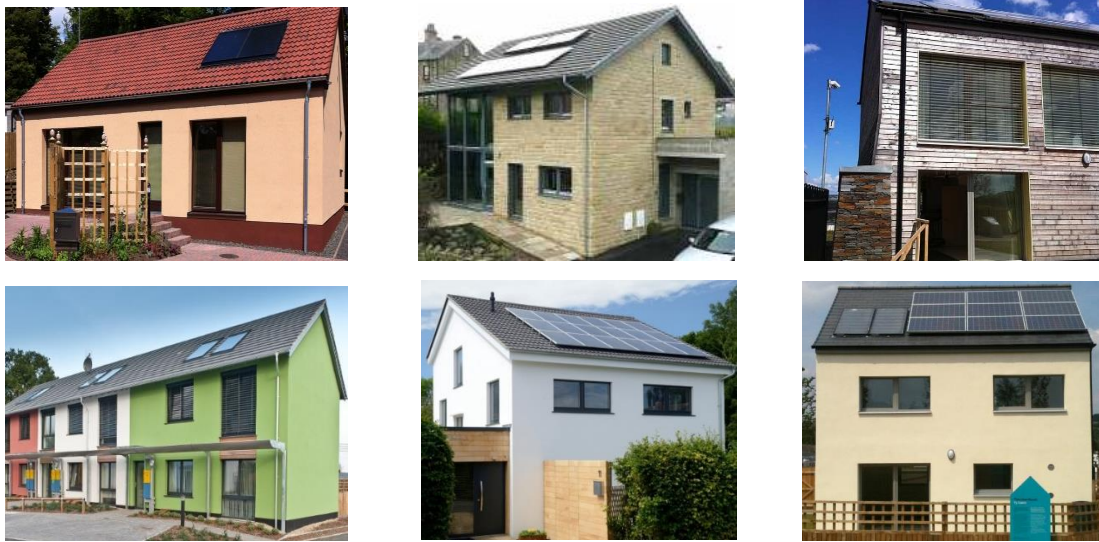
Figure 1-2 Examples of UK Passivhaus: clockwise from top left Sunnyside Passivhaus, Denby Dale Passivhaus, Larch House, Wimbish Passivhaus, Totnes Passivhaus and Lime House
