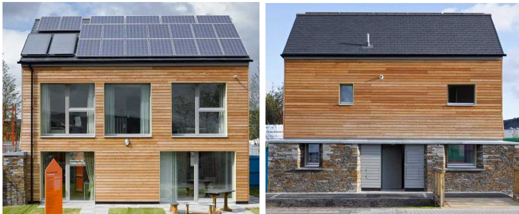
Figure 5-2 South (left) and North (right) elevations of the Larch House
