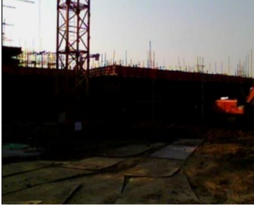
(c) Optical image with poor lighting condition
