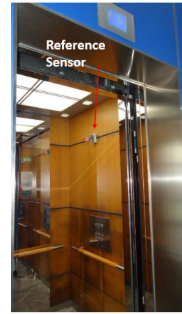
(f) Fixed reference node installed in the lift
