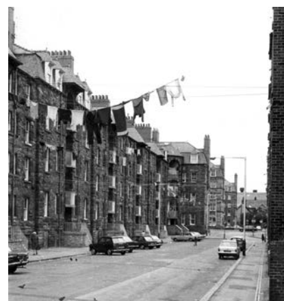
St Martin's Cottages facing demolition towards the end of their working life in 1968.
