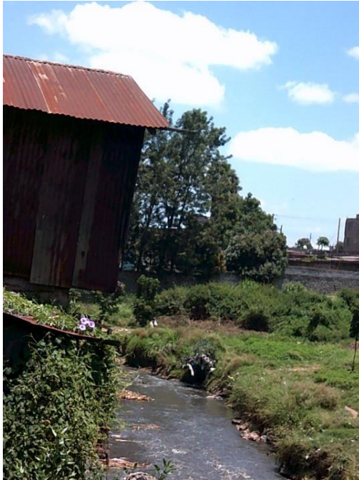
Photo 23 Unstable housing located overhanging river
