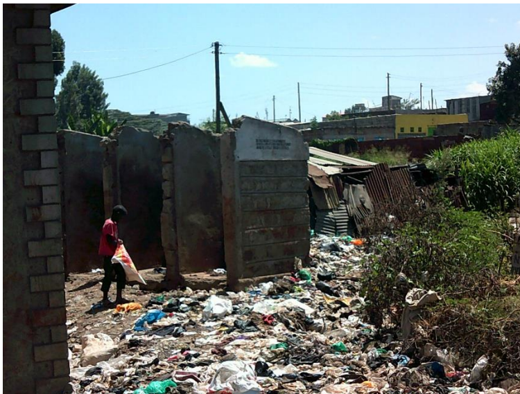
Photo 21 Toilets without doors identified as high risk location for rape
