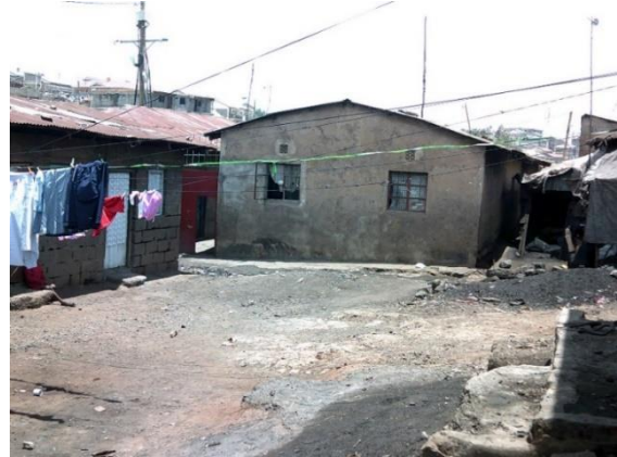
Photo 22 Safe and clean enclosed compound
