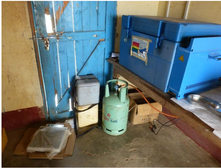
Photo 5 Gas cylinder for refrigerator at remote health facility
