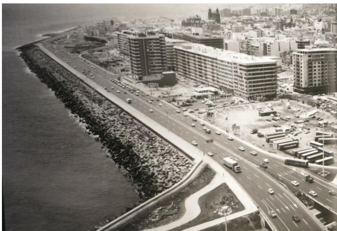
Figure 18 - Infrastructure Las Palmas ca. 1980
