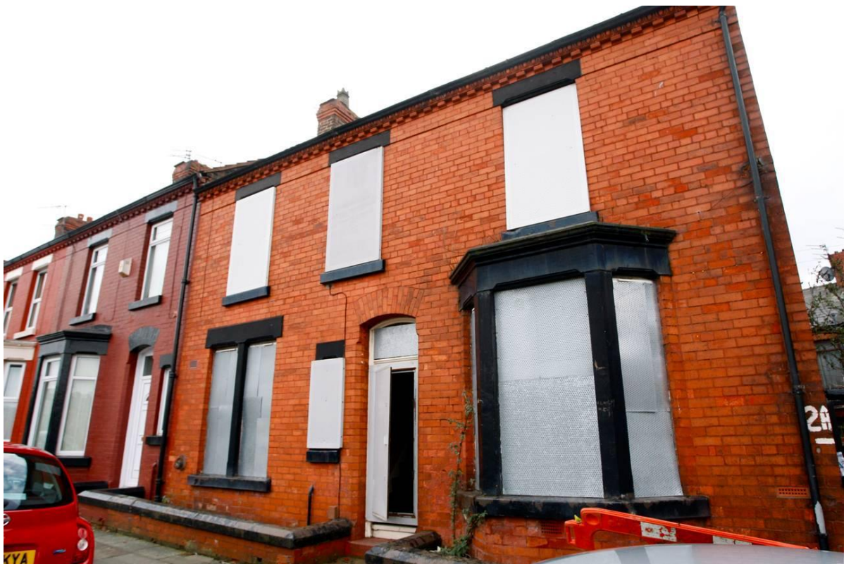
Figure 0:1: 2 Broxton Street House before retrofit
