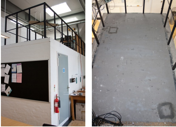
Figure 14: The concrete floor of a small transmission suite was used as receiver structure for Case Study 2. The floor has dimensions of 2.1 m \times 3.1 m and is approximately 130 mm thick. It is supported by masonry walls on four sides and can therefore not be considered a “free” plate as required for the reception plate method.
