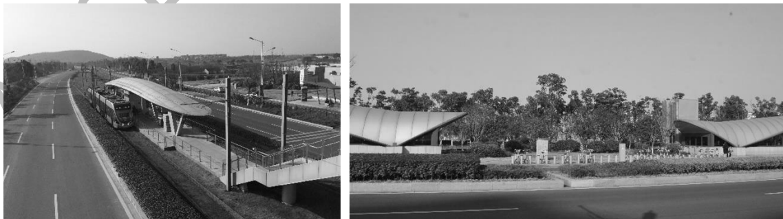
Figure 16 Access to the SND tram: examples of an overpass bridge ( left ) and underpass tunnel ( right ).
