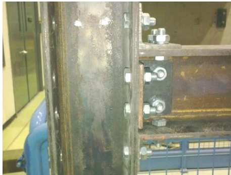
(c) Beam-column connection on the left hand side of the first storey
