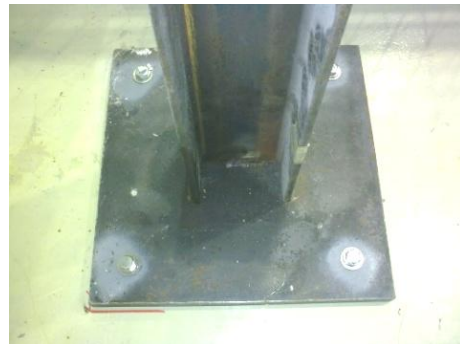
(f) Column-base connection on the right
