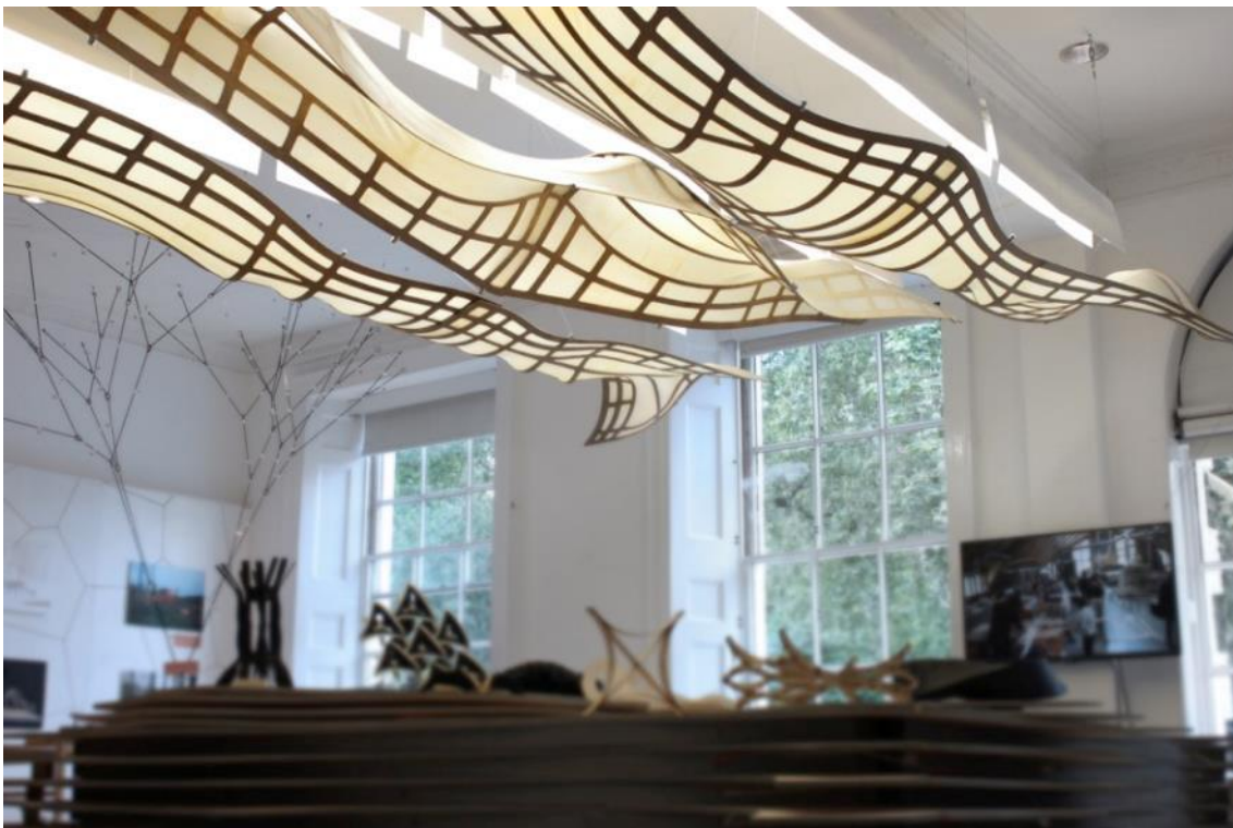
Figure 10: Real scale plywood composite components serving as suspending ceiling (photo by the authors)
