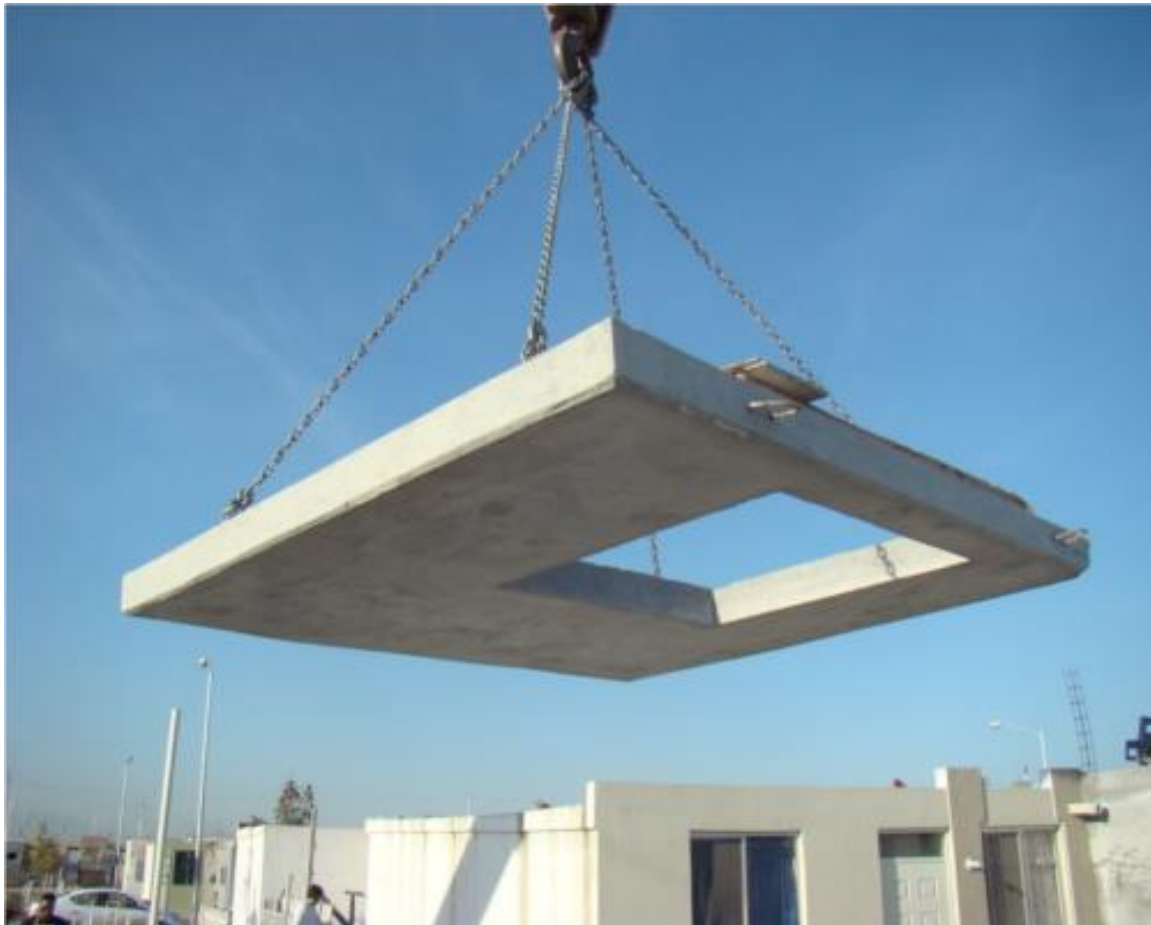
Figure 3.4 Installation of a prefab roof slab (Grupo GIC, 2016).
