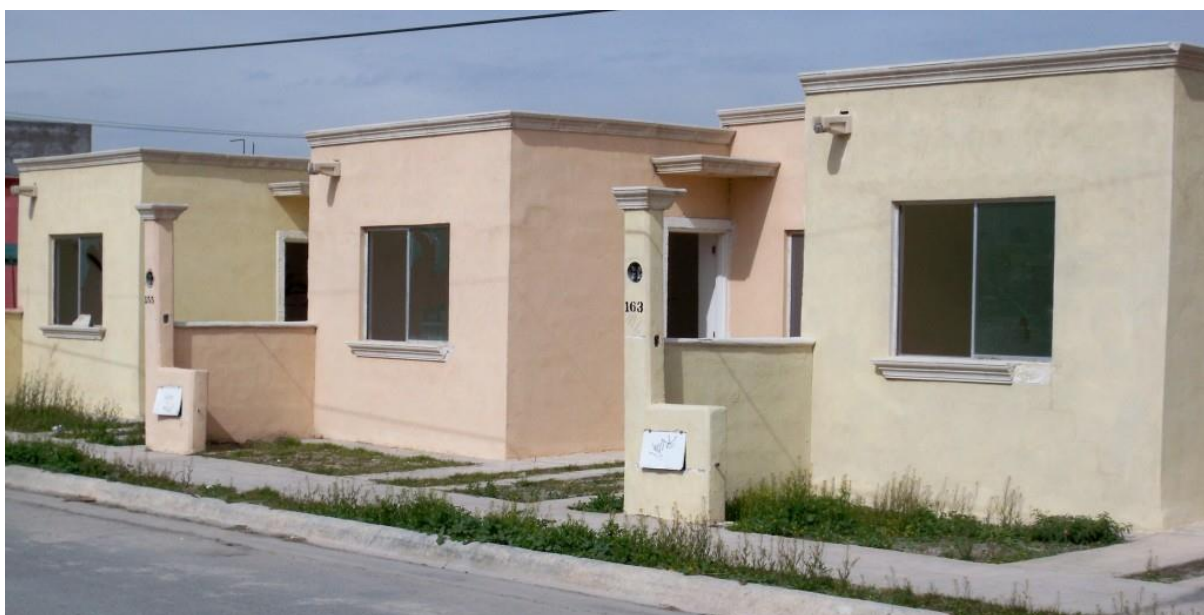
Figure 2.6 Row house social housing facade
