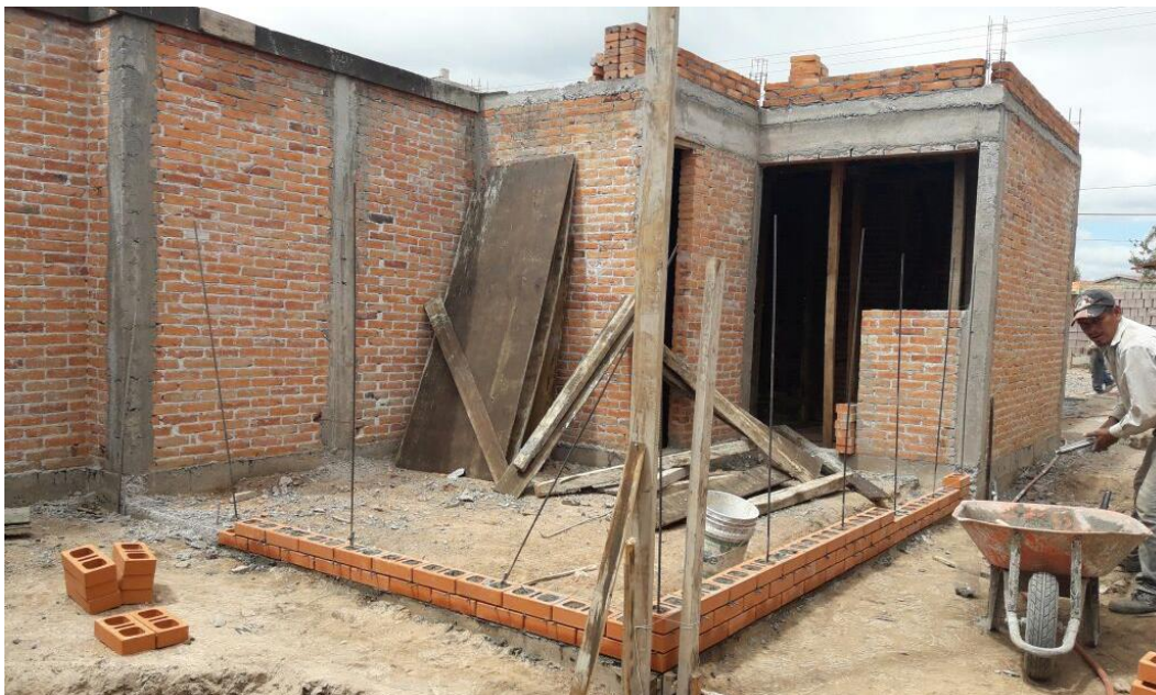
Figure 3.3 Traditional construction system.
