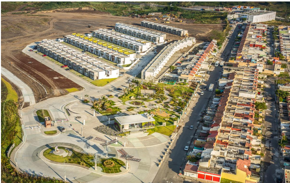
Figure 2.12 shows the stark contrast between the traditional densely packed social housing neighbourhoods (right) with the open areas and wide streets from ALIKA (left). (Anon., 2017)
