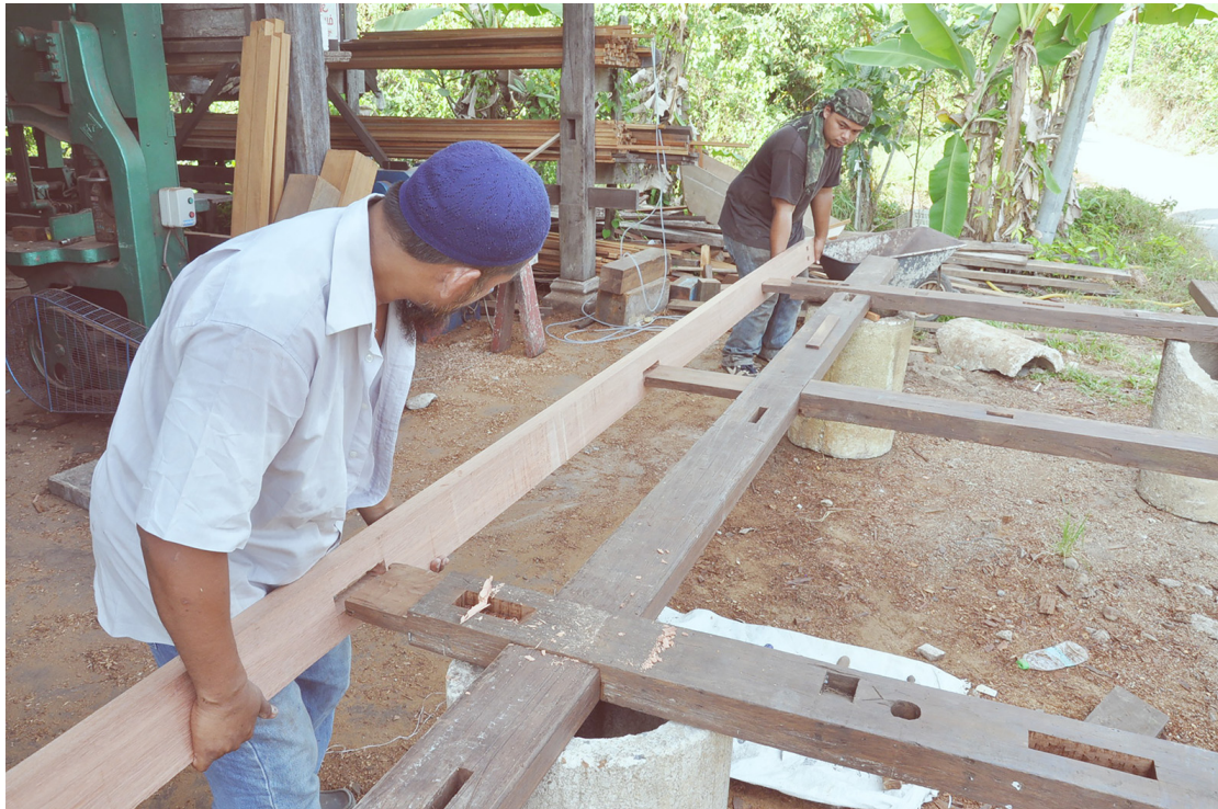
Figure 4: Modern Malay tukang with his young apprentice installing the timber component in the assembly of a roof structure prior to construction on-site.
