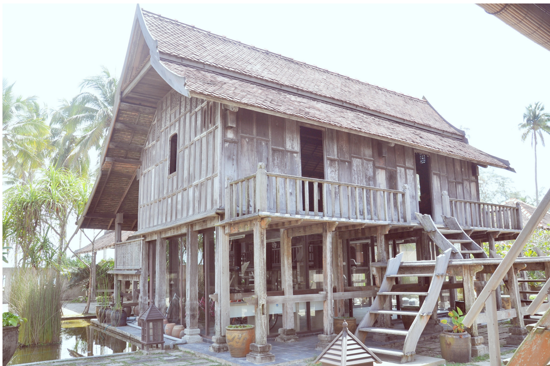
Figure 1: Example of a traditional Malay house in Terengganu with a regional variation of form and style influenced by Thai architecture. This structure was disassembled, reconstructed and restored as a resort building in Terrapuri heritage village.
