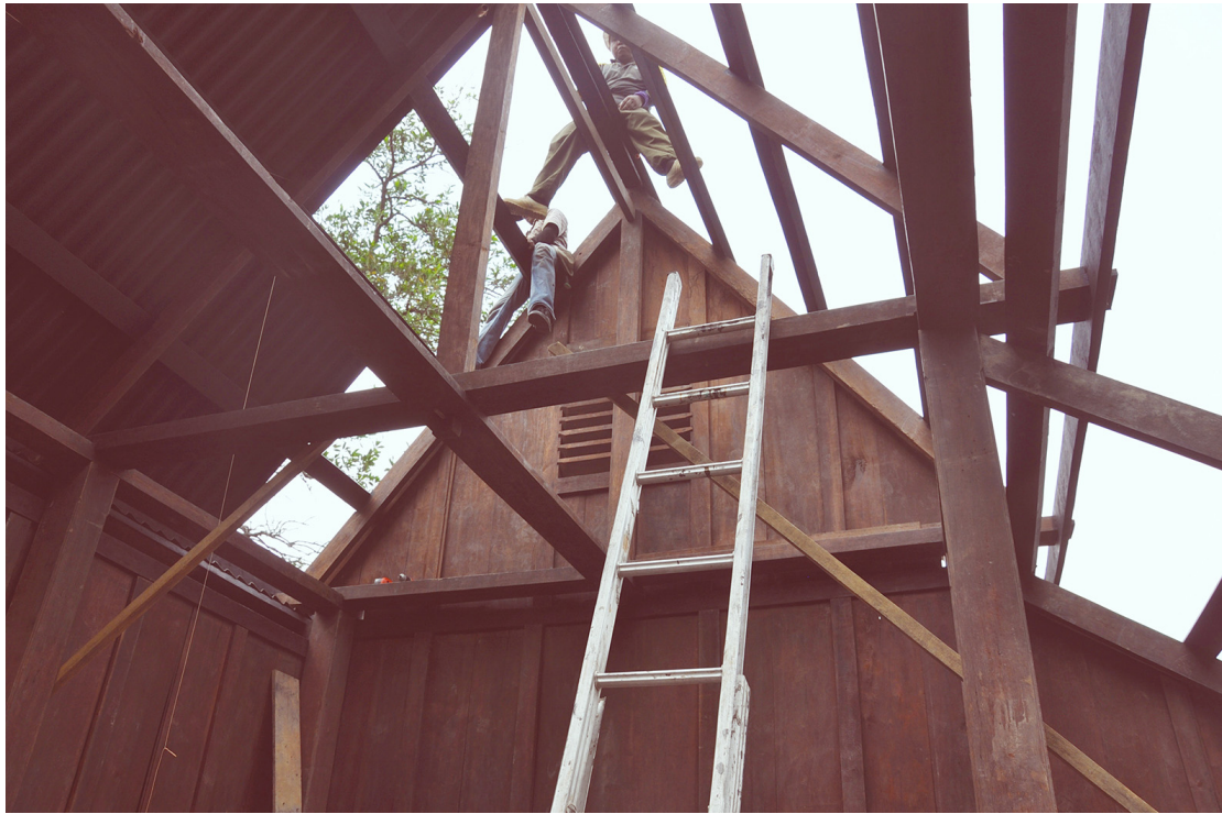
Figure 8: This ninety year old traditional house was disassembled from Pahang and re-assembled in The University Putra Malaysia, Selangor, as a conservation exercise coordinated by the Malay Heritage Museum. The reconstruction includes the use of modern day material as part of the roofing element.
