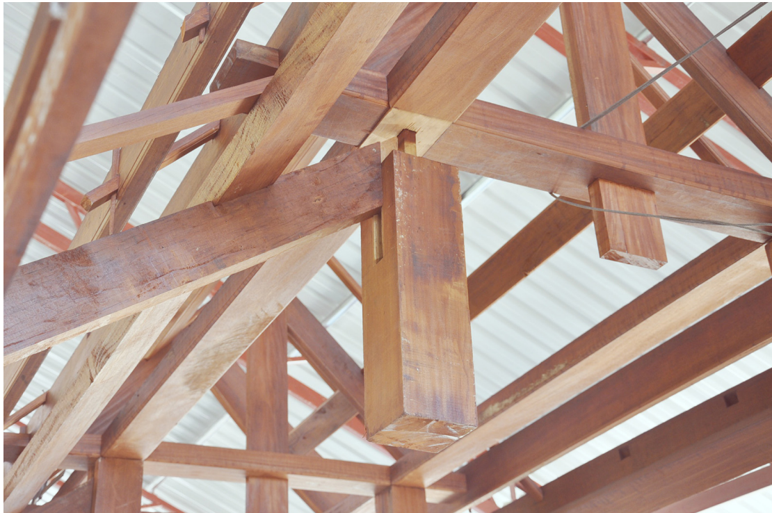
Figure 9: The disassembly and assembly process requires the understanding of procedural techniques as each building components are assembled based on sequential order.
