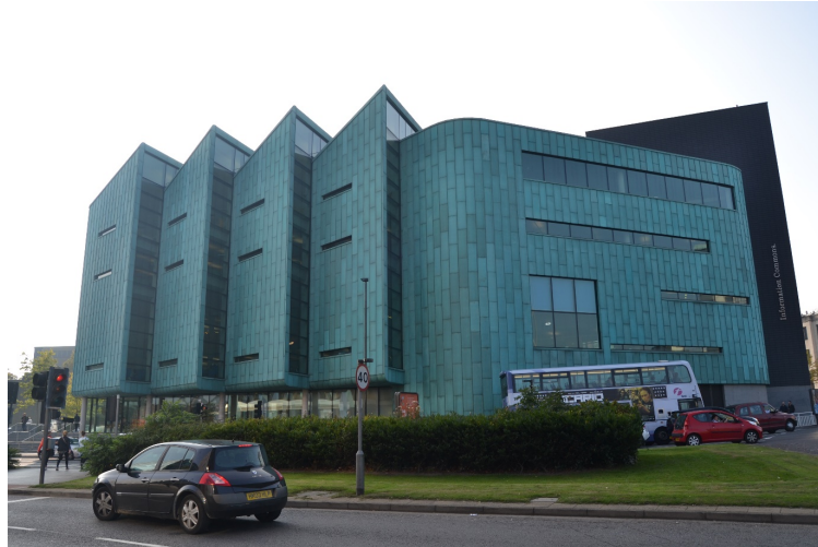
Fig. 9. External view of the Information Commons.
