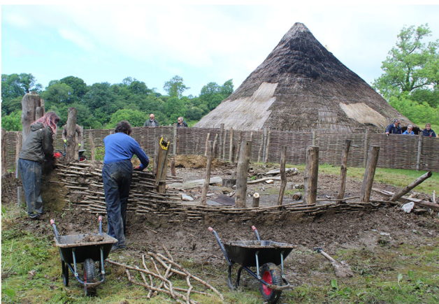
Fig. 13 Partially standing Cookhouse wall with wattle and daub and slumped wall materials
