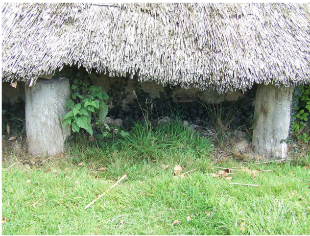
Fig. 9 Cookhouse Phase 4 wooden rafter props set on flat stones
