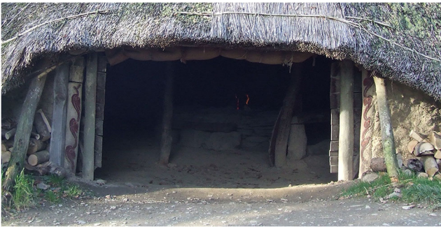
Fig. 27 Earthwatch roundhouse doorway modifications supporting the decorated original door jambs, taken 2017; note the naturally-formed eaves drip gully across the threshold
