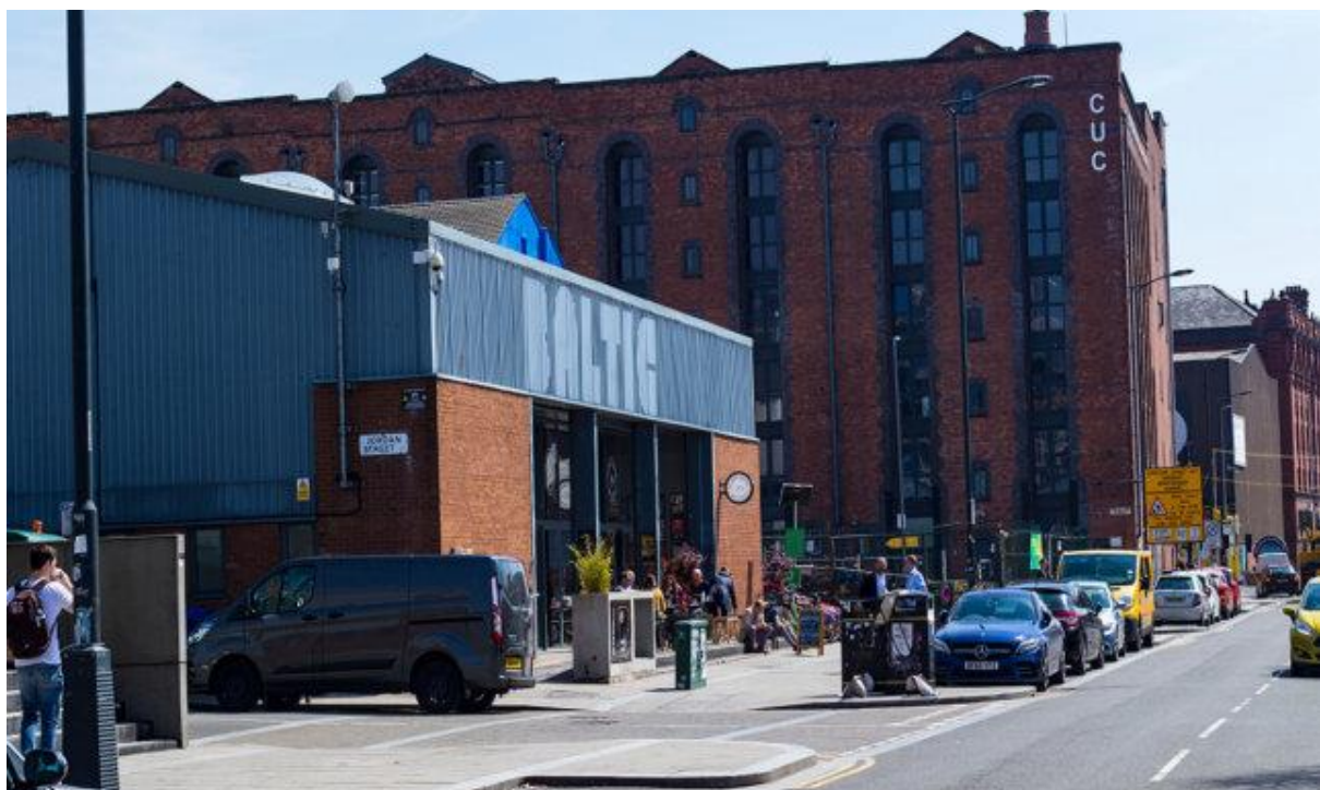
Figure 9: Image of Sub-Demo Area A showing industrial buildings repurposed into creative businesses and housing (Jessett, 2019)
