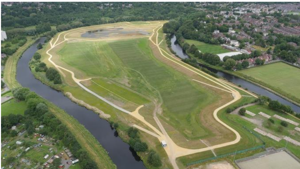
Figure 4: Urban wetland created as part of £10 million Salford Flood Scheme (Environment Agency, 2018)
