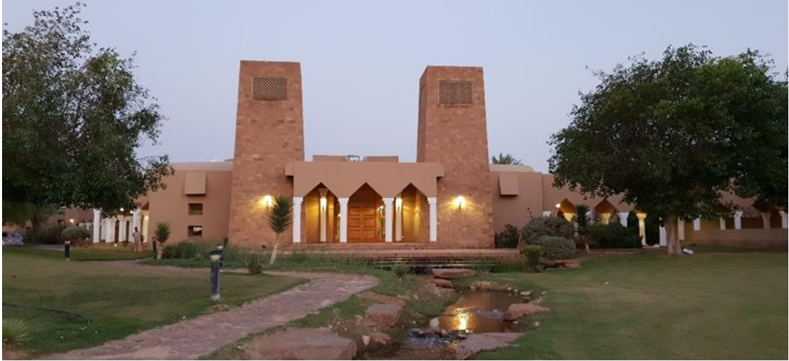
Figure 4-1: The main entrance of Dar Al-rhmaniah Library and the two cooling towers
