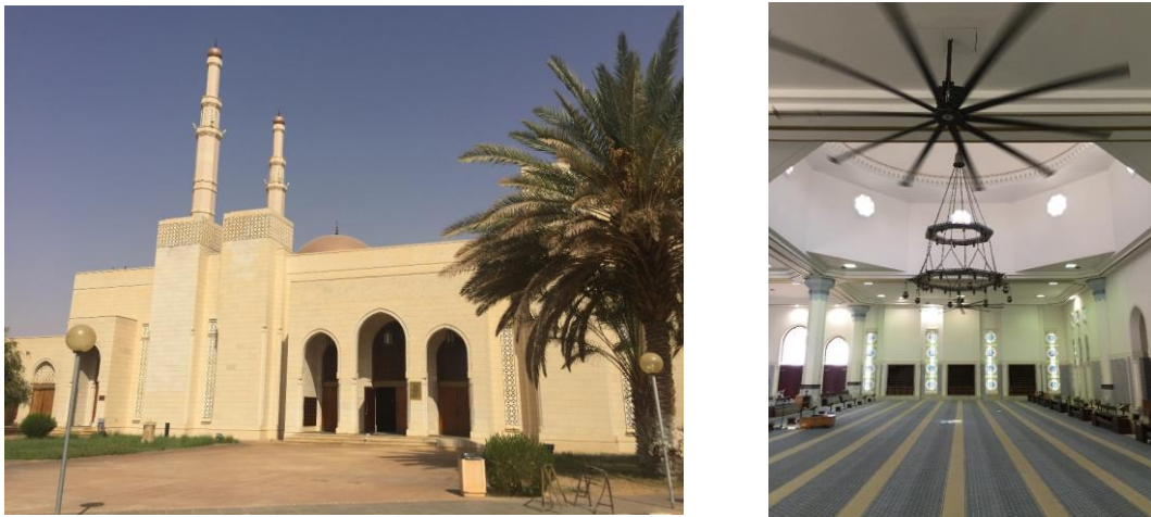
Figure 3-5: External and internal pictures of Al-Rahmania mosque showing the cooling towers and supply openings
