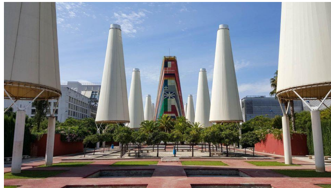
Figure 3-2: PDEC (Shower) towers at Seville EXPO'92
