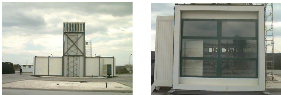
Figure 5-2 Experimental PDEC tower built in Catania (Galatà and Sciuto, 1997)
