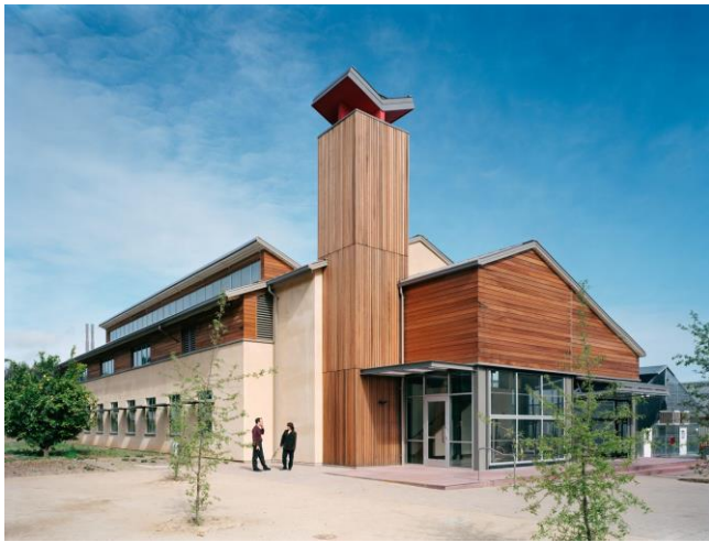
Figure 3-13: External view of the GERCC showing the PDEC tower (CBE, 2020)
