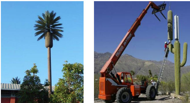
Fig.1. Base station antennas on camouflage platforms.
