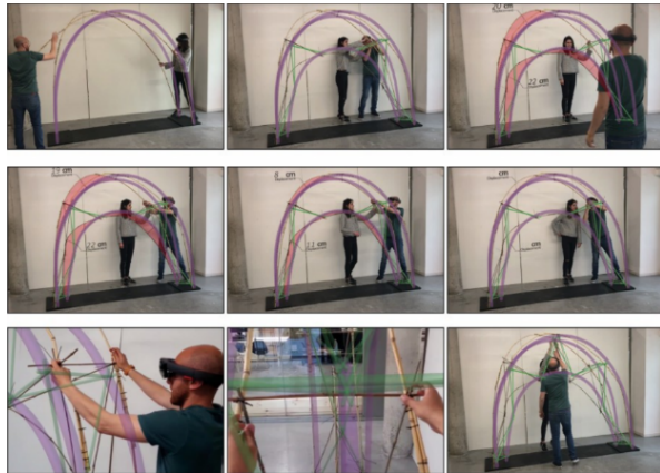
Fig. 15: Cyber-physical construction process in AR. This figure was produced by A.Akbari from IAAC programme Master in Advanced Architecture in 2018 [36], and it summarized that during the fabrication, the differences between 3D virtual blueprints and the physical structure are constantly monitored and the user tried to follow the virtual guide as much as uncertain behavior of the material allows in AR. The permission to re-use the figure has been granted by the author and the publisher.
