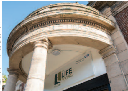
Fig 7. The Walton Life Rooms building's defining central dome was retained and emphasised because of its uplifting quality, and 'because it did not remind people of the sanitised, detached quality typical of healthcare facilities'.
