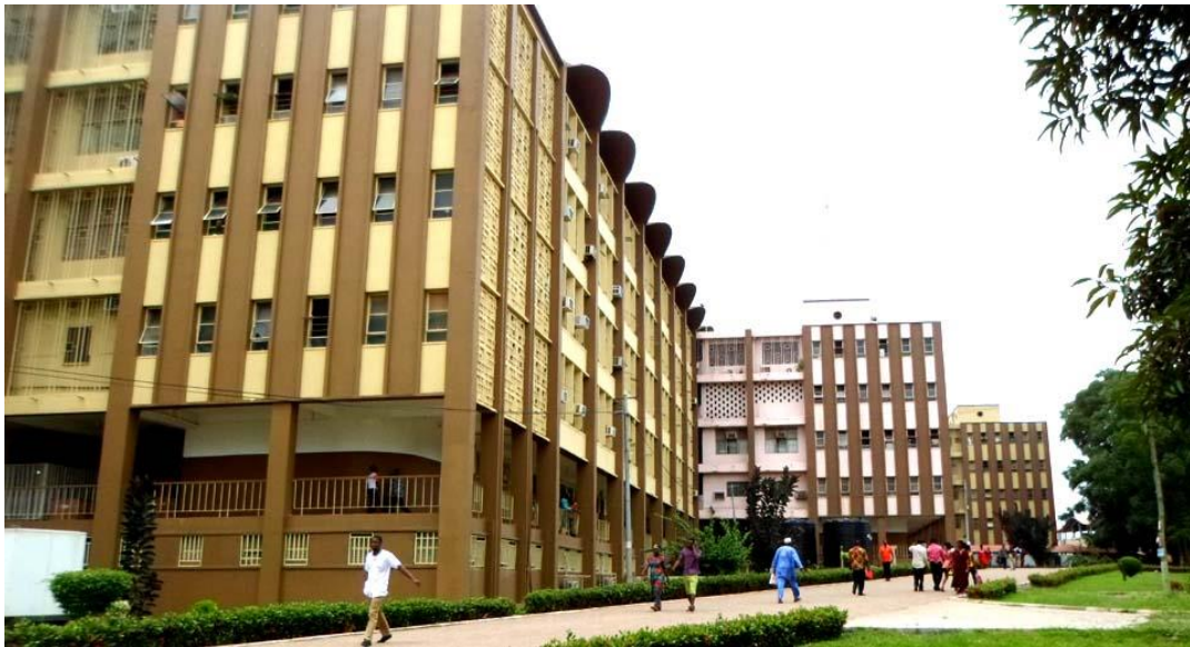
Figure 1. 4: The side view of the Komfo Anokye Teaching Hospital building
