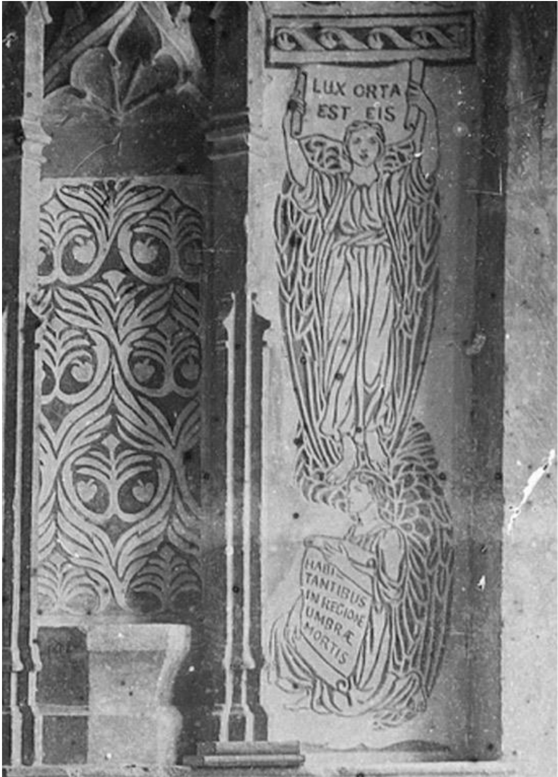
Fig. 5: Detail of right-hand side of east wall in figure 4, showing Sumner's mature style of sgraffito virtually fully developed, (Neg. ref. C3-113). The text is from Isaiah, second half of verse 9.2. The first half was in the panel to left of the altar. The full Latin text reads: 'populus qui ambulabat in tenebris vidit lucem magnam habitantibus in regione umbrae mortis lux orta est eis' (The people walking in darkness have seen a great light; on those living in the land of deep darkness a light has dawned).
