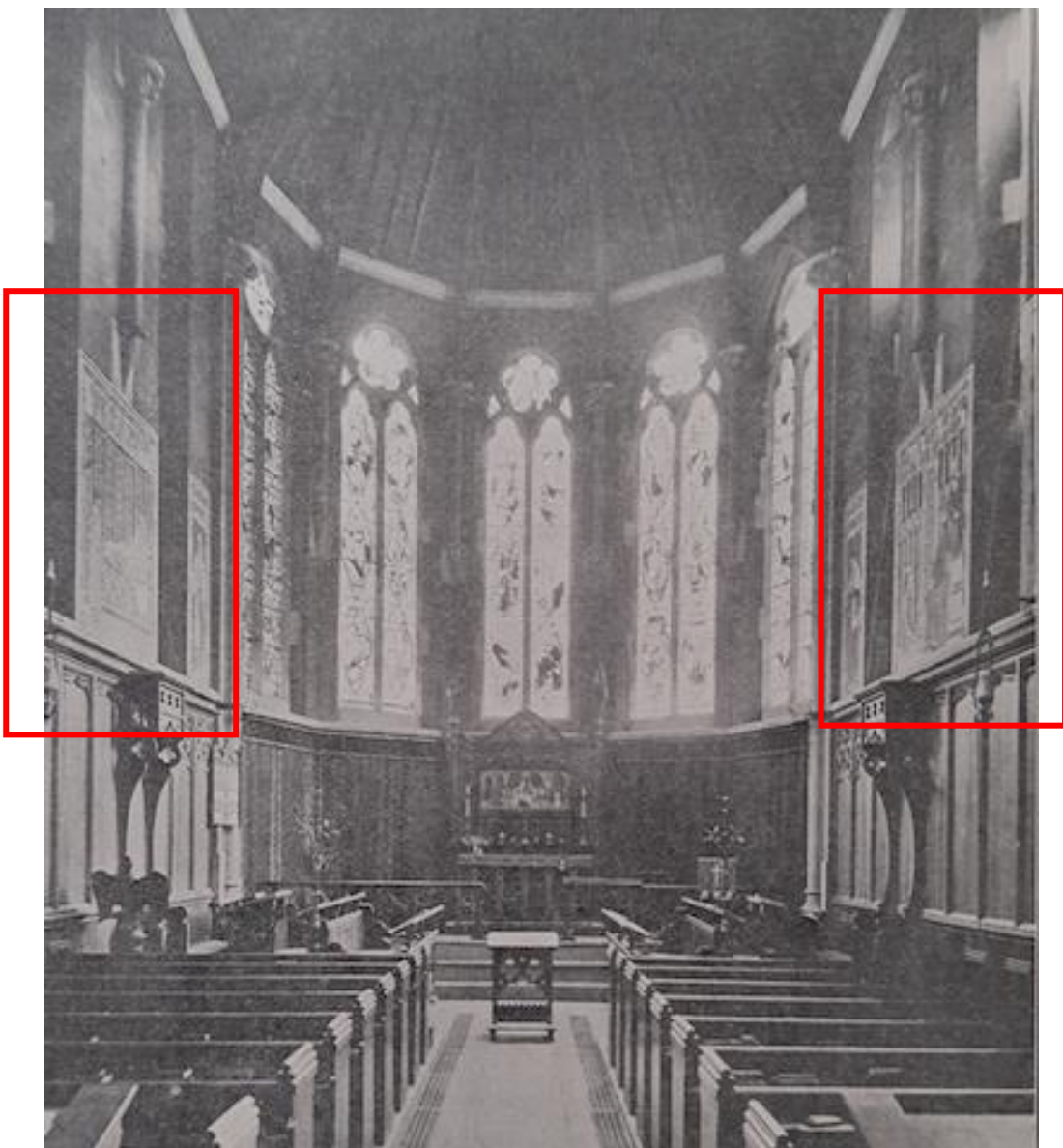
Fig. 2: Interior in 1903 with sgraffito panels outlined in red on left and right walls above panelling.
