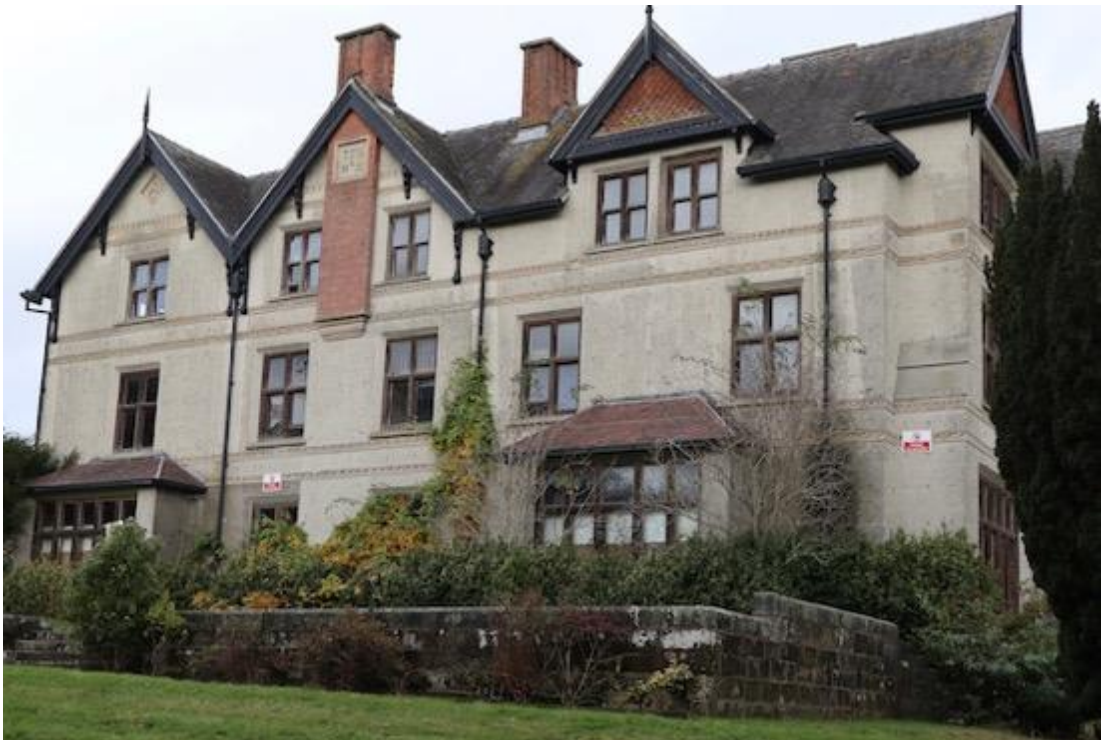
Fig. 4: South front in 2020. The string courses are incised decoration probably either stamped or done using templates as work in Devon churches was. The gable plaques give, on the left, the date 'AD 1875' and the initials of Thomas Percival Heywood, the second baronet, and his wife, Margaret (it is assumed), 'TPH & MH.'
