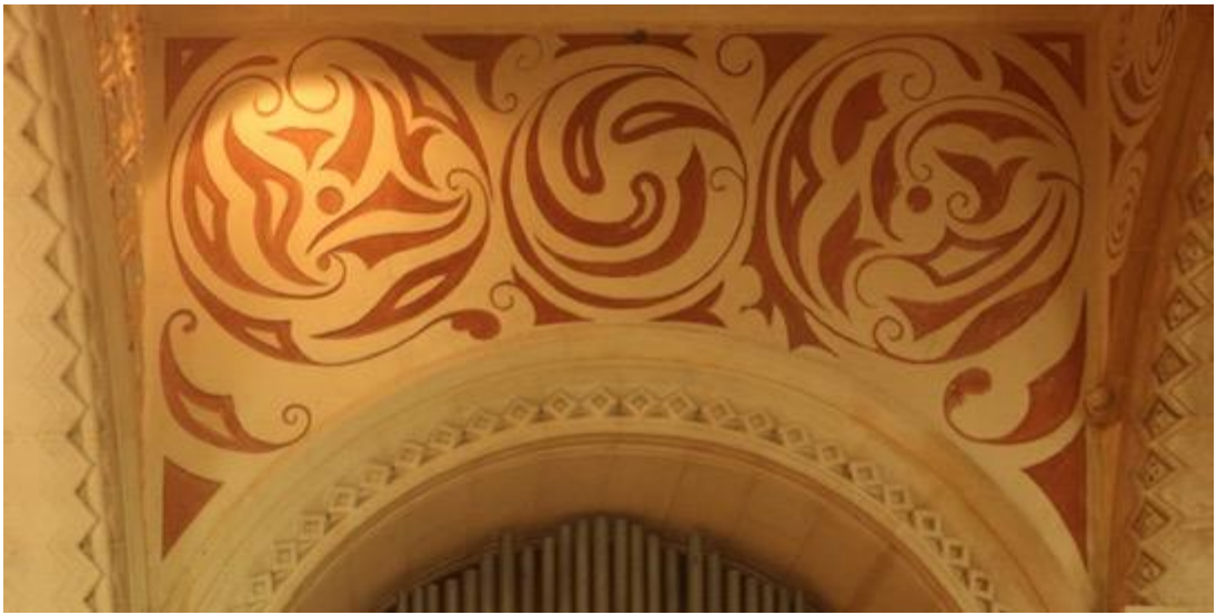
Fig. 6: Sgraffito over the north transept arch, which also occurs on the chancel arch to the right.
