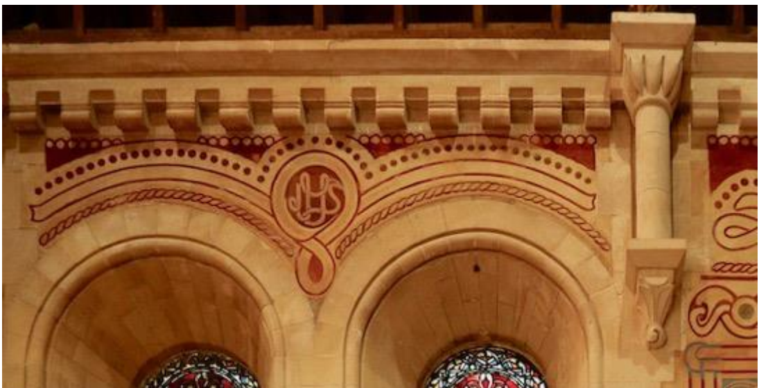
Fig. 4: Sgraffito over the north chancel windows with a monogram abbreviation at the centre for the name of Christ.
