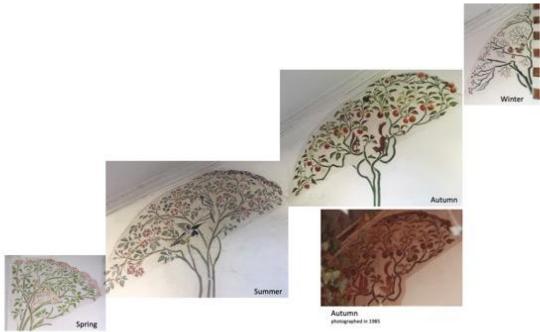
Fig. 9: Hill House. Four Seasons composite elevation as existing, with comparison photograph from 1985, showing evidence of overpainting.
