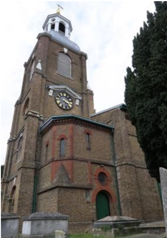
Fig. 2: Teulon's extension to the south aisle, delicately fitted if slightly awkward.
