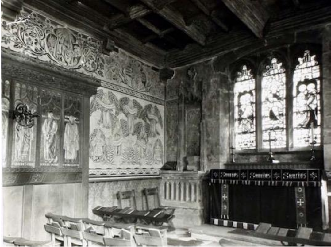
Fig. 8: 1943 interior view looking north-east. This view is similar to figures 4 and 6 but turned so as to show more of the north wall, and the figure of the prophet Jeremiah top left. (Historic England, 5249/2 or 004).
