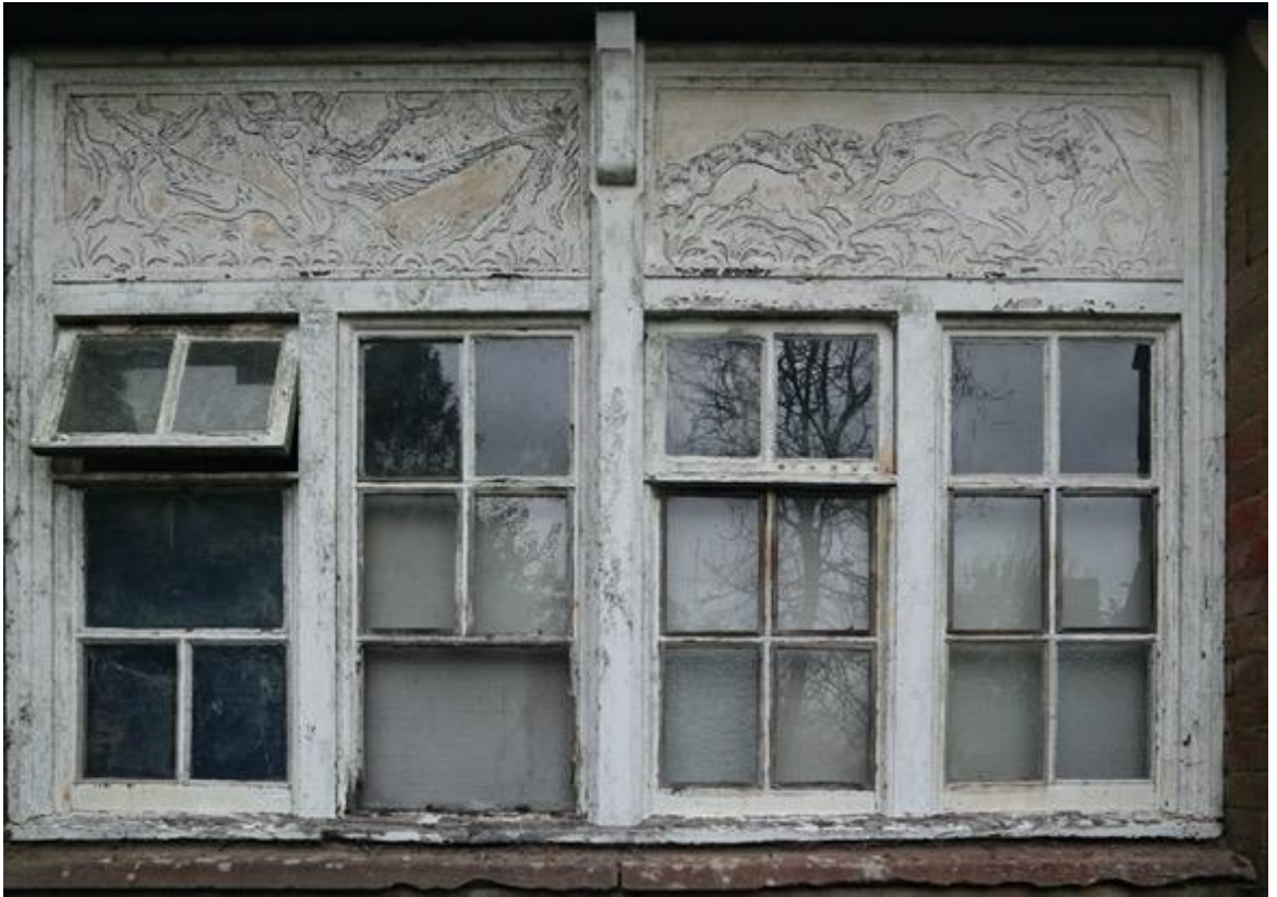
Fig. 16: Window frame setting of panels 1 and 2.
