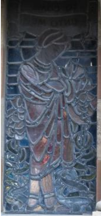
Fig. 40: Window in figure 39 seen from outside showing the strong and complicated lead line structure.
