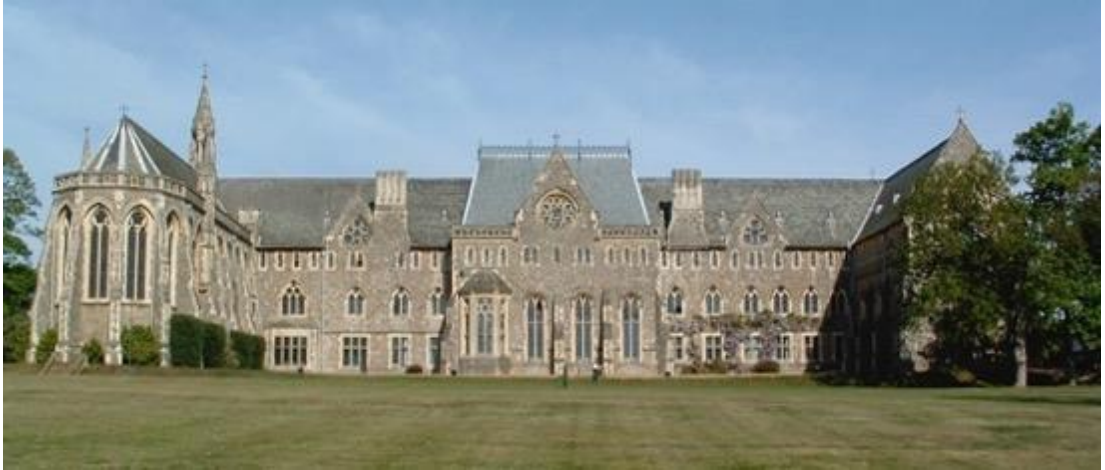
Fig. 1: Southeast front of school with chapel to the left.
