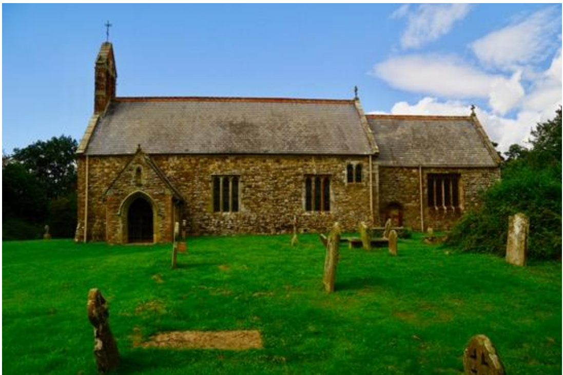
Fig. 2: St Mary's. South elevation.
