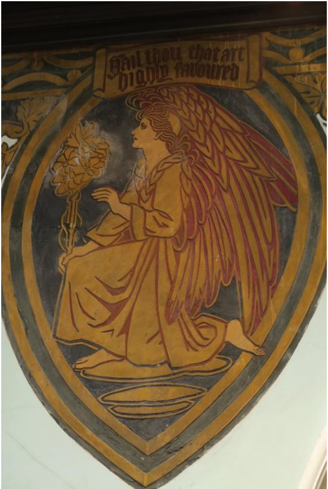
Fig. 7: South. The angel at the Annunciation, 'Hail thou that are highly favoured'. Note the salt damage from water penetration round the lily and the way the angel's foot breaks the picture boundary.
