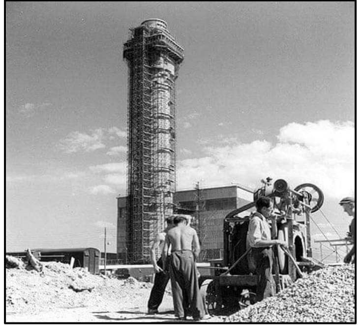
Fig 7.0: Construction of the first Windscale pile, July 1950. (Sellafield Ltd)
