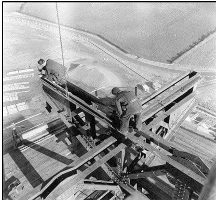
Fig. 8.0: Construction workers atop Windscale pile number one, c. 1948. (Sellafield Ltd)
