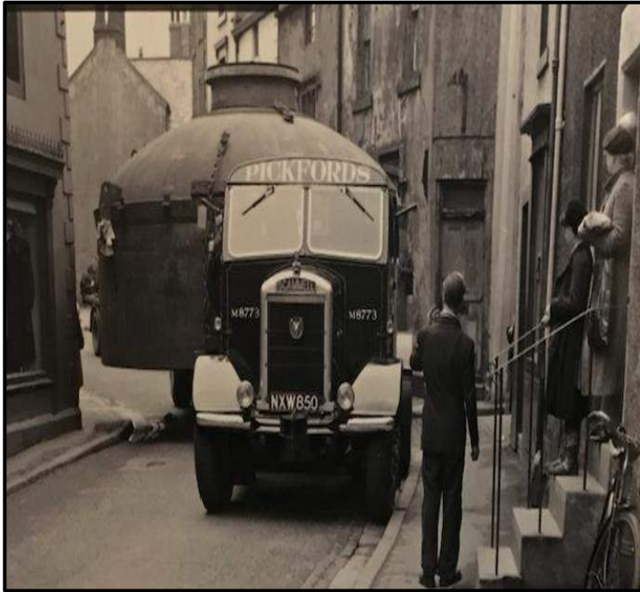
Fig. 6.0: Heat exchanger passing through Egremont. With kind permission from the Beacon Museum, Whitehaven.
