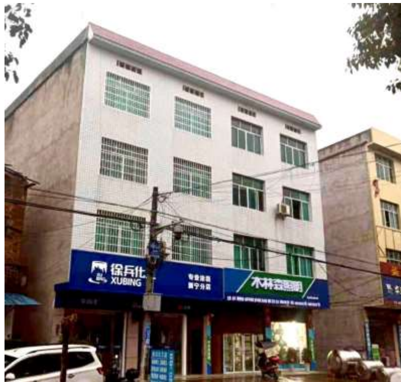
Figure 3-2: View of case building (semi-detached dwelling on the right).
