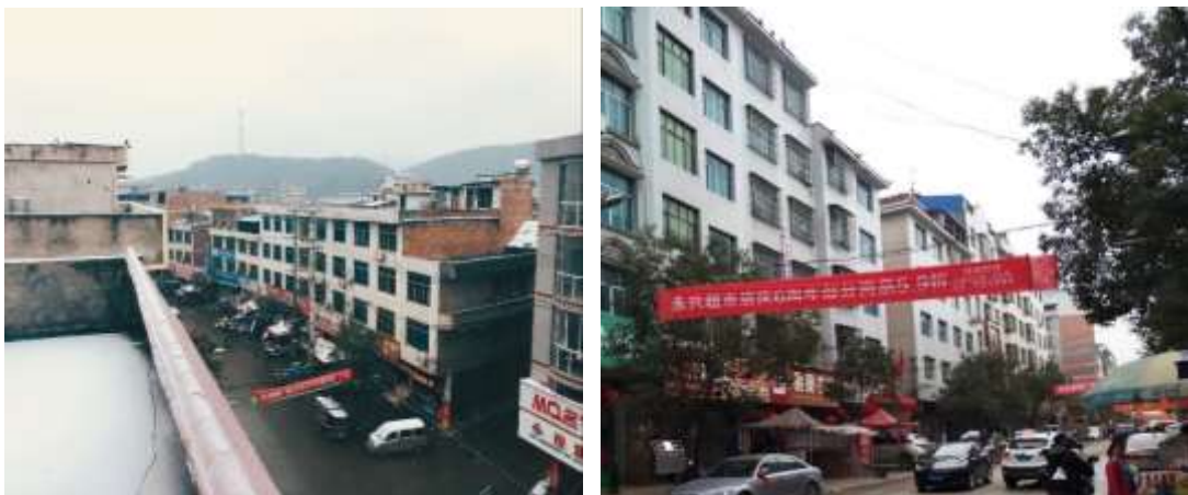
Figure 2-7: Town (suburban) residential buildings in Hunan province.
