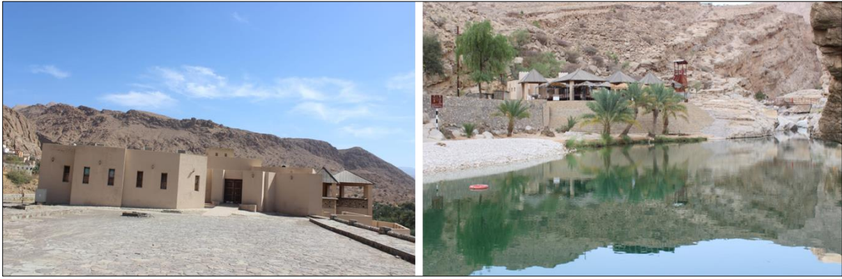
Figure 30: The unused visitor centre in Muql village (left) and the coffee shop building in the pools area (right) (pictures taken by the researcher on 29 July 2018).
