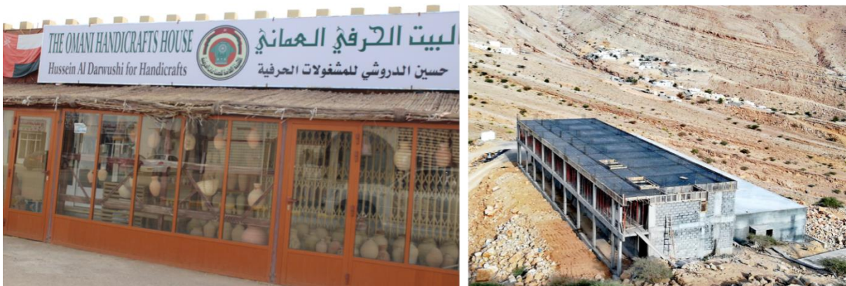
Figure 71: The Omani Handicrafts House in the centre of Wadi Bani Khalid on the way to Muql village (left) and the guest house under construction in Muql village (right) (pictures taken by the researcher on 28 July 2018).
