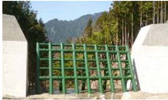
Figure 3. 4 (left) a solid closed rock check dam (Vente 2007). Figure 3. 5 a open steel slit check dam located at Sabo Dam (Mizuyama, 2008).
