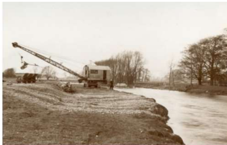
Figure 1. 1 maintenance along the River Dove in the 1940s using a drag line to remove woody debris and create a trapezoidal channel. Source Mott, 2010
