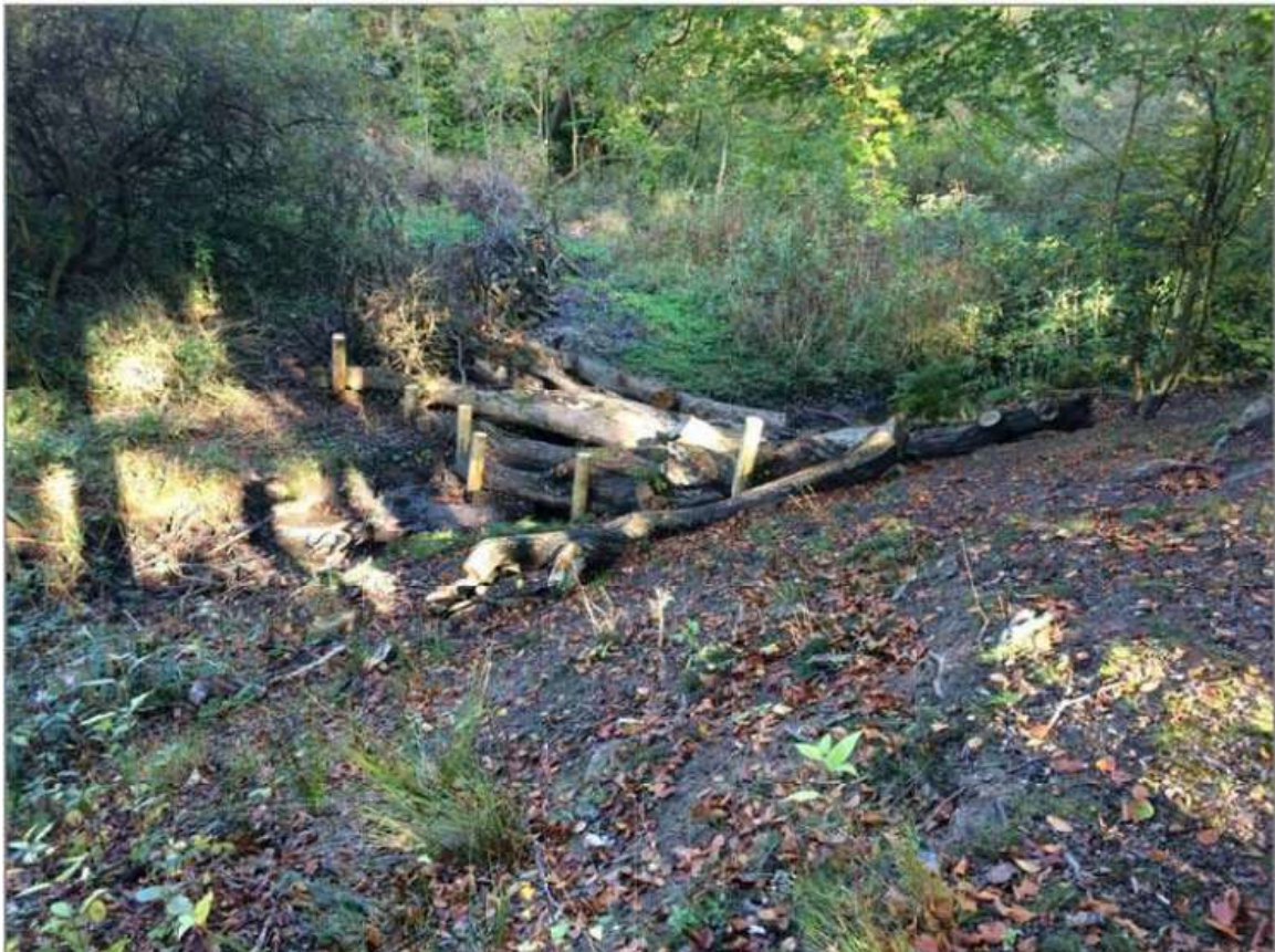
Figure 5. 2 LWD constructed along the Stanley Brook. Photograph was taken from the top of the valley. The LWD can be seen to extend across the vegetated floodplain.
