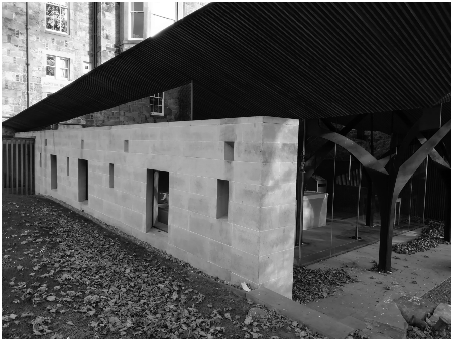
Figure 31.2 Case study building exterior view – St Albert the Great chaplaincy, Edinburgh (G. Treacy)
