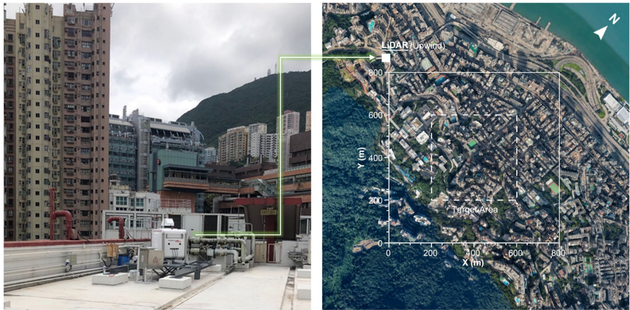
181 182 Fig. 2. The selected high-density urban site (800 m × 800 m) in Sai Wan, Hong Kong for reproducing vertical wind 183 speed profiles, and the wind LiDAR location on top of the roof of Yam Pak building (15 m above the ground). 184
