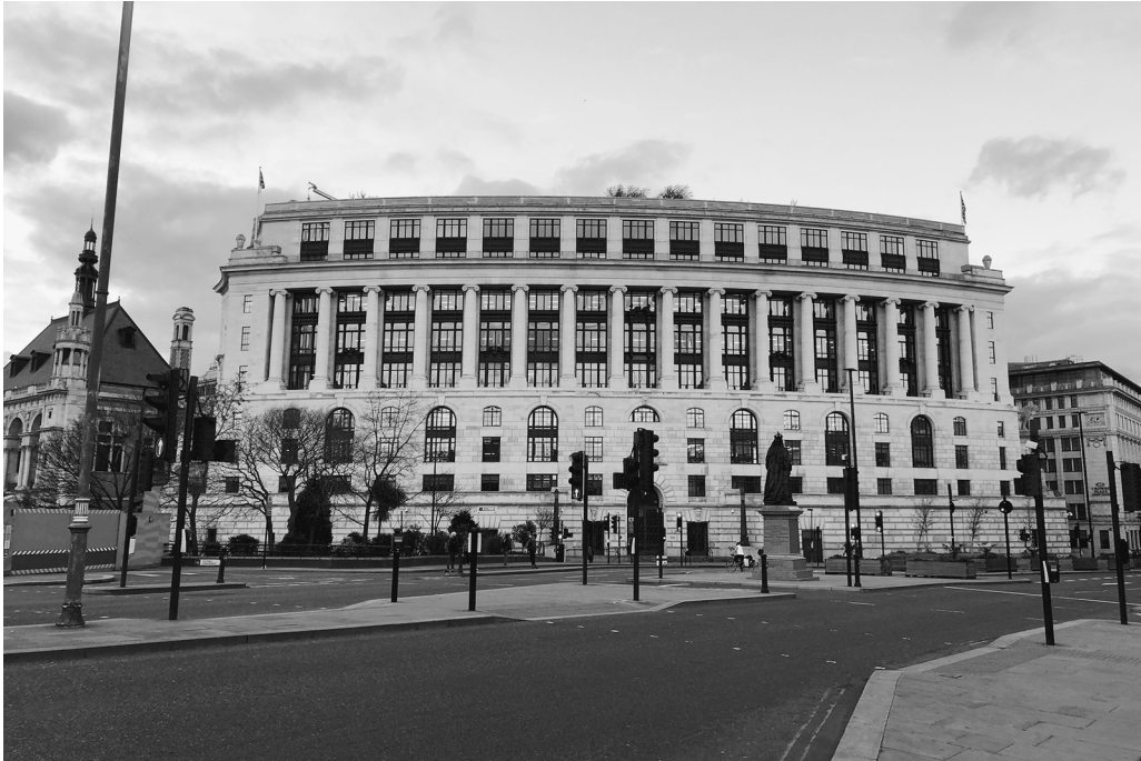
Figure 1. View of Unilever House, 2021. Photo: Author.
