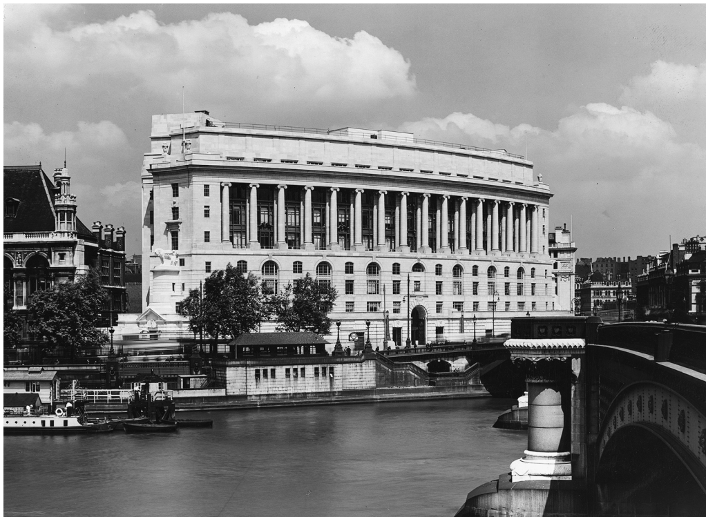
Figure 3. Unilever House in 1932. The top of the building was a blank wall and not used as office spaces. Photo: RIBA Photo Library.
