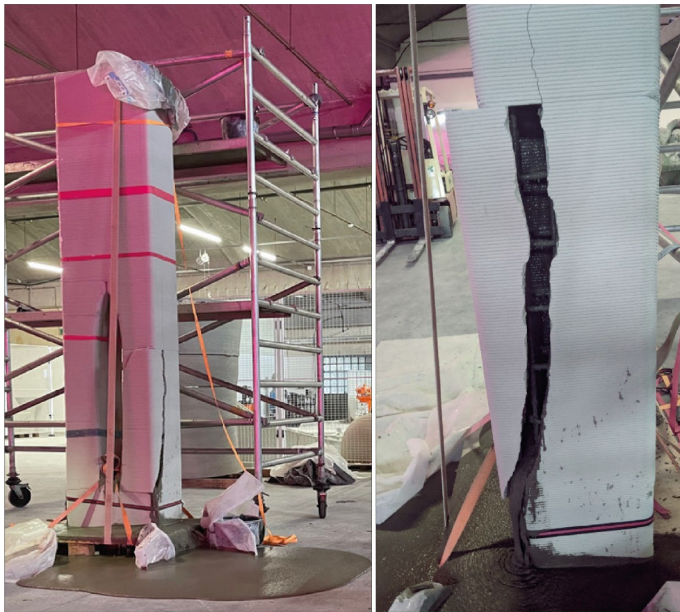
Figure 30: Failure of casting due to the hydrostatic pressure on the 3D printed formwork
