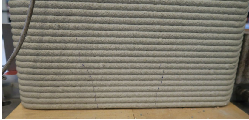
Figure 34: Small cracks appeared on the printed surface of the 1:2-scale prototype after applying a load test of 80 kN
