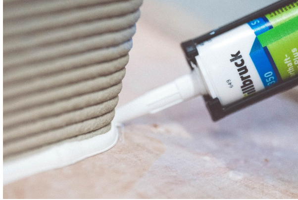
Figure 24: Adhering the 3D concrete printed formwork before casting with self-compacting concrete
