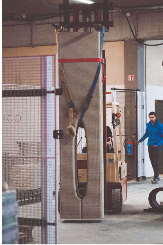
Figure 21: Transporting the column using straps attached to the centre hole of the column
