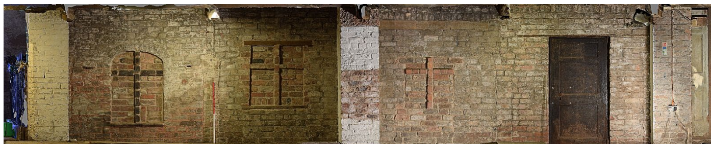
Figure 8. Photogrammetric image of the burial vaults in the crypt after the entrance blockings had been reinstated, with Vault 1 on the far left and Vault 4 with the cast iron door on the far right.
