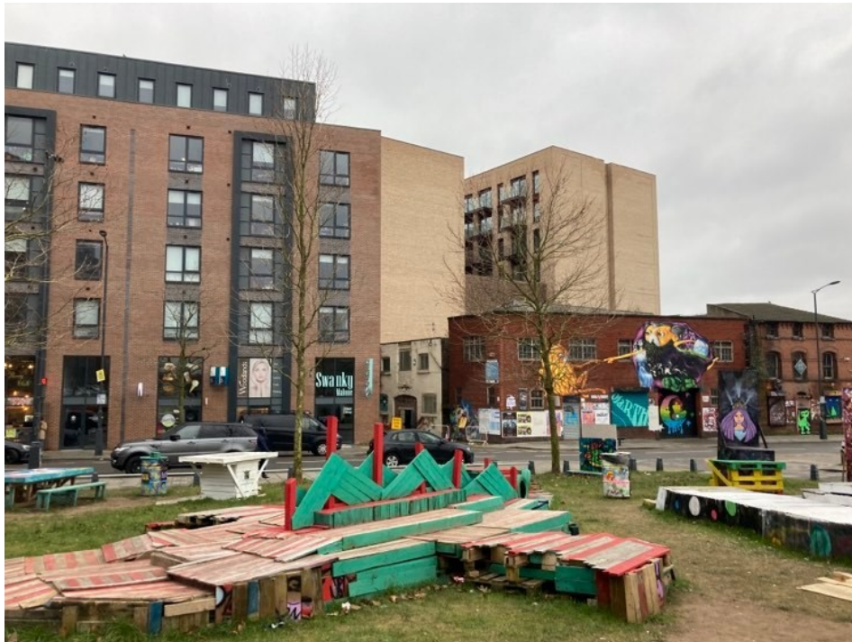
Figure 4.12 24 Kitchen Street (tiny white building), viewed across the green, surrounded by neighbouring developments now completed
