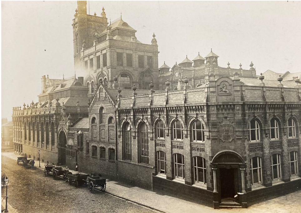
Figure 1.5 The Cain's brewery, shortly after completion in the early nineteenth century
