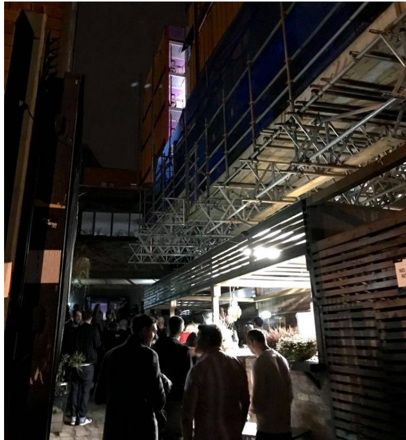
Figure 4.11 24 Kitchen Street courtyard with the imposing scaffolding of neighbouring development in-progress
