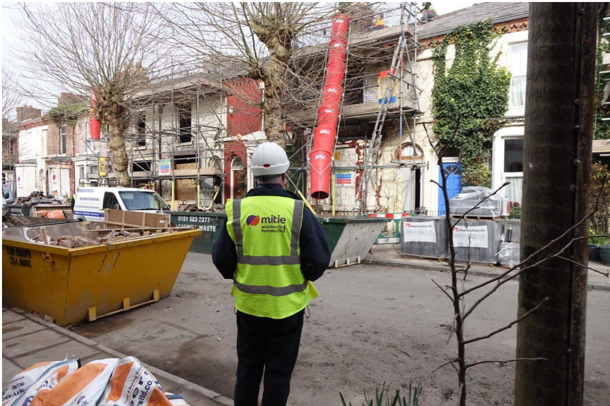
Figure 27. Contractors Mitie onsite.
