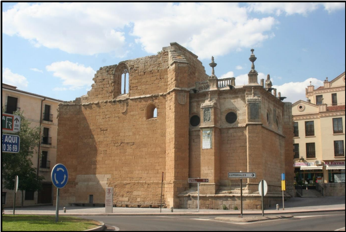
Figure 25. The remains of the San Francisco convent. (Photograph taken by the author August 2015).
