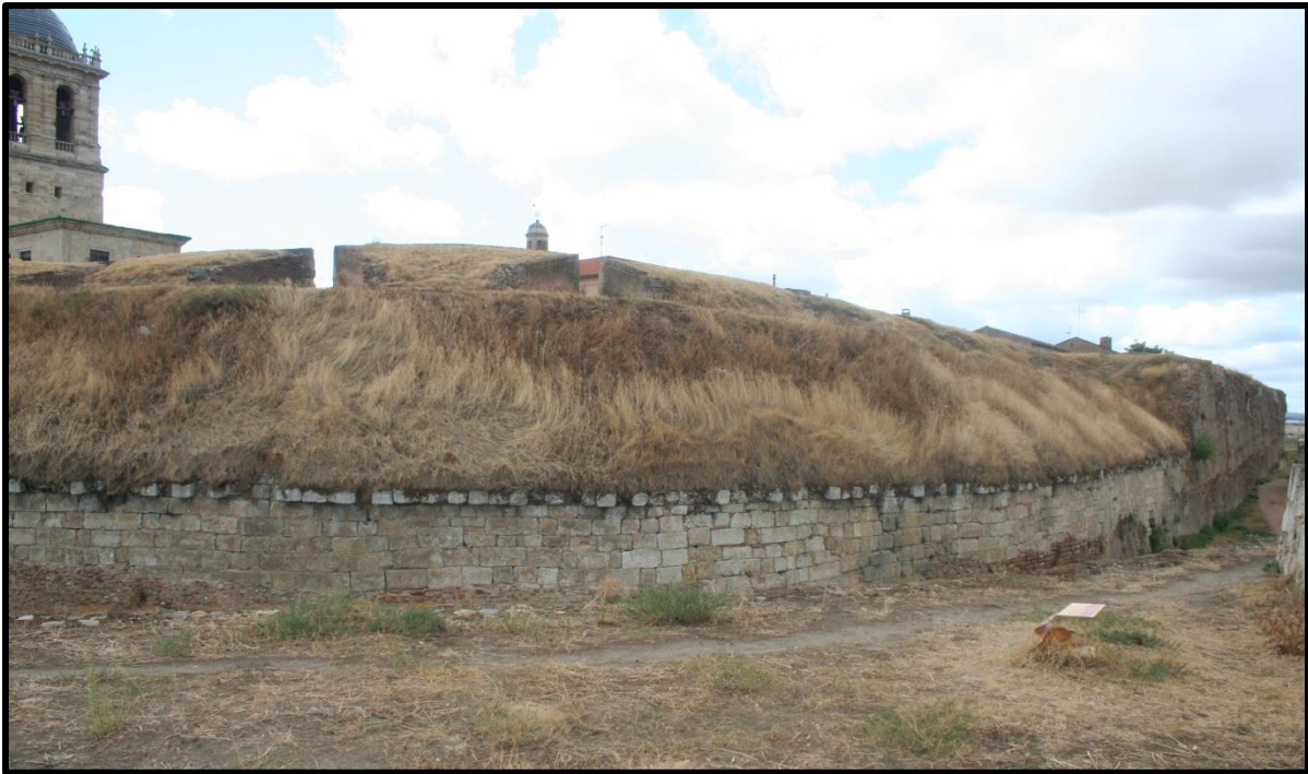
Figure 12. Site of the 'Great Breach' at Ciudad Rodrigo. (Photograph taken by the author August 2015).
