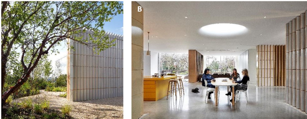
Figure 6-5: Maggie's Southampton a) the reflective stainless-steel surface behind the ceramic wall, b) polished concrete floor.
