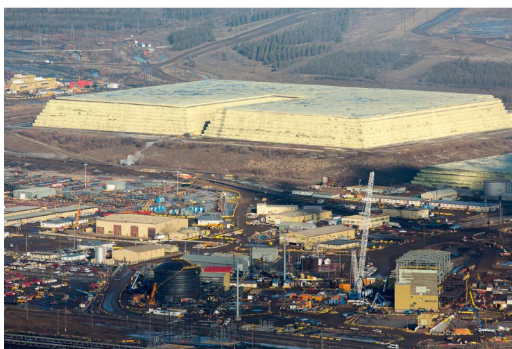
Figure 1.6: Photograph of the large blocks of sulfur, a by-product of crude oil refining at the Syncrude Mildred Lake site, Alberta, Canada. 18 Credit: Alex MacLean
