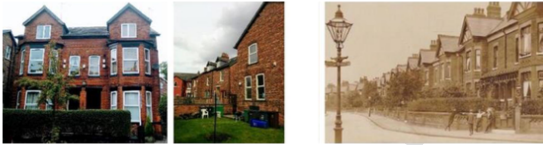
Fig. 1. The Zetland Road Victorian townhouses pre-retrofit [43].
