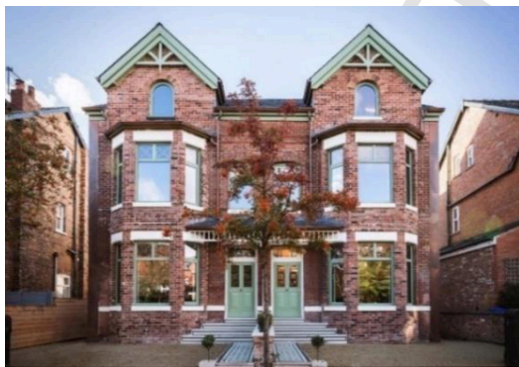
Fig. 2. Zetland Road Victorian townhouses after refurbishment [43]- colour should be used in print.
